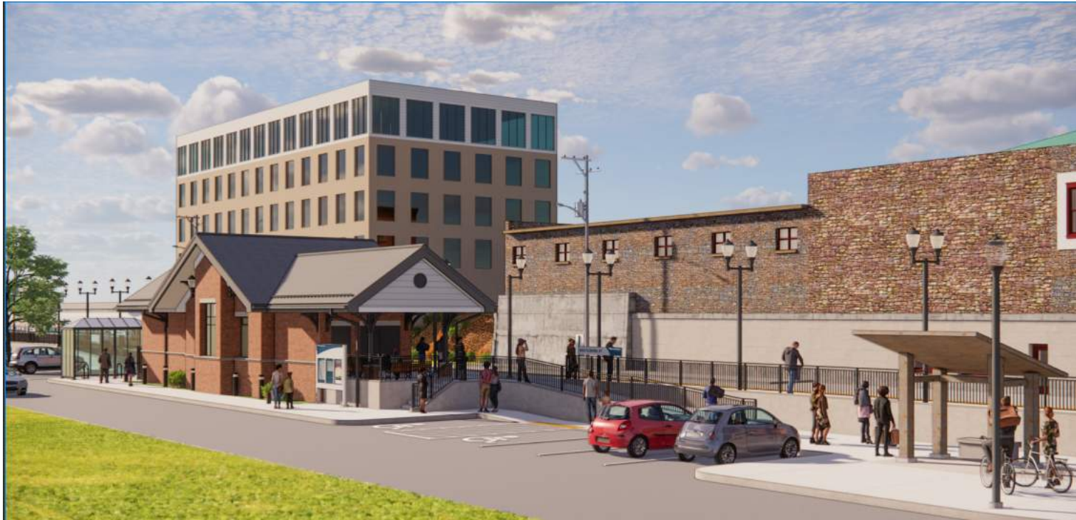
View of site looking south towards the new station building
