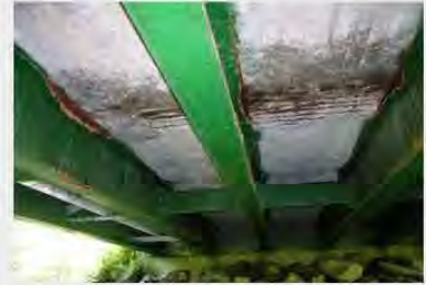
Deck Deterioration
