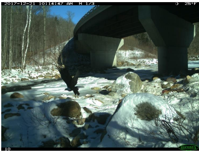
Bald eagle at span 9-25b, Searsburg
