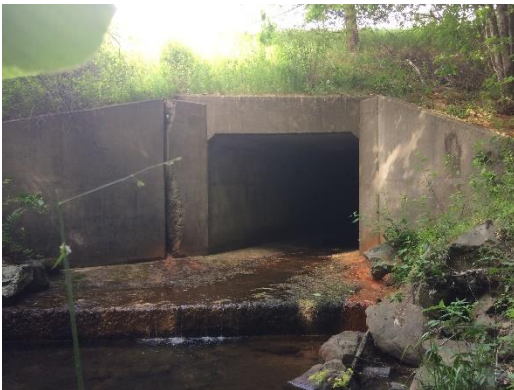
Figure 29. Example of a V bottom box culvert , with “dry concrete” movement surfaces along culvert walls. Site I91-17-2, Putney.
