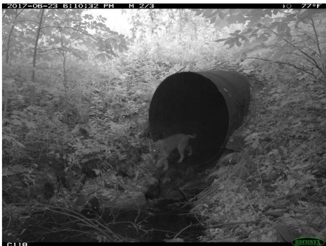
Bobcat at pipe culvert in Manchester (Site 7-19-5)
