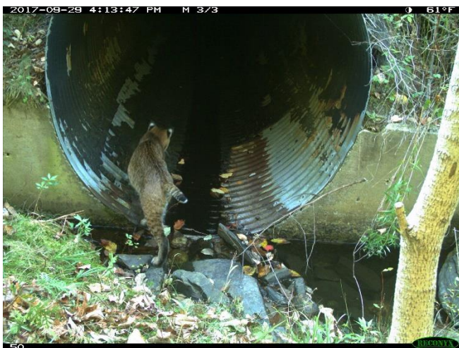
Bobcat at pipe culvert I91a, Sheffield
