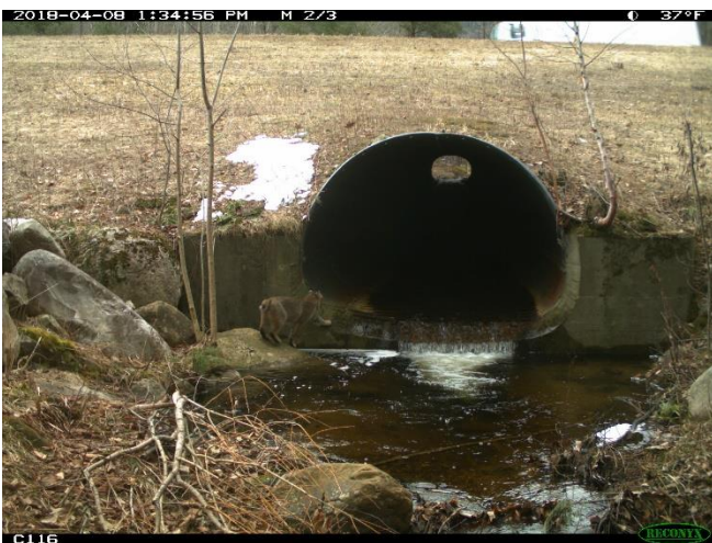
Bobcat at squash pipe 7-19-5, Sunderland
