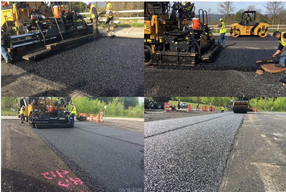
Figure 5: Open Graded Friction Course Paving
