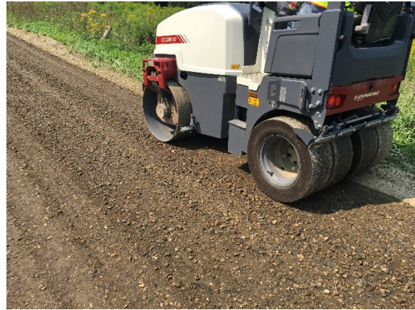
Two passes of the 2 ton roller
