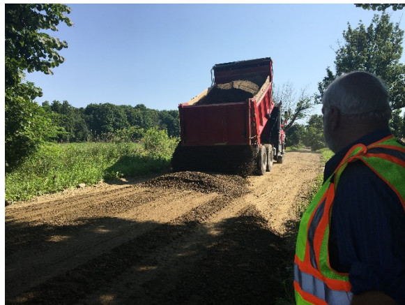
Truck dumped and spread material
