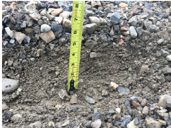
Segregation of material
