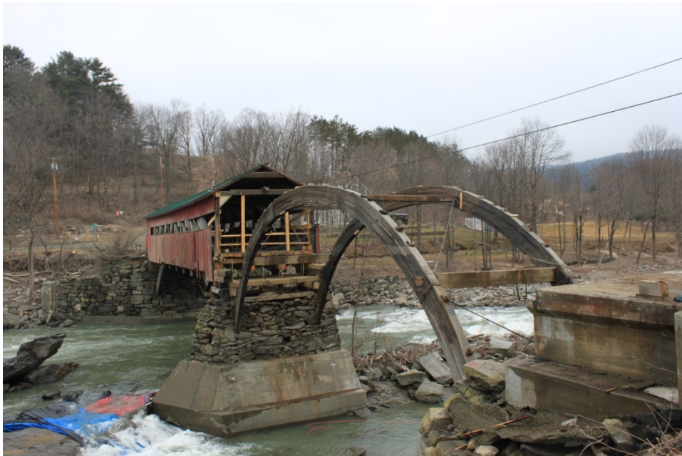
Figure 10: Western span dismantled leaving only the arches
