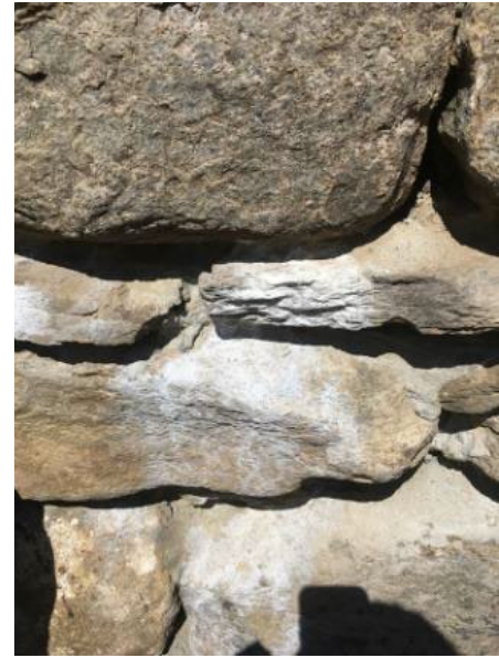
Figure 18: Southern Abutment and closeup of mortar leachate (2017)
