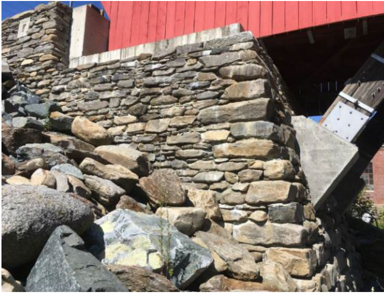
Figure 18: Southern Abutment and closeup of mortar leachate (2017)
