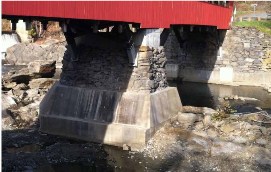
Figure 16: Completed pier showing the concrete cap and abutment
