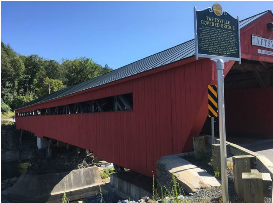
Figure 3: Taftsville covered Bridge after repair in 2012
