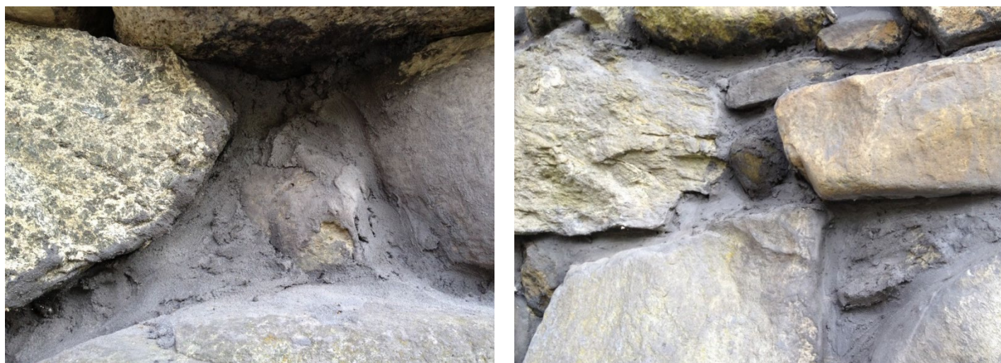
Figure 14: Up-close view of stone pointing and mortar work
