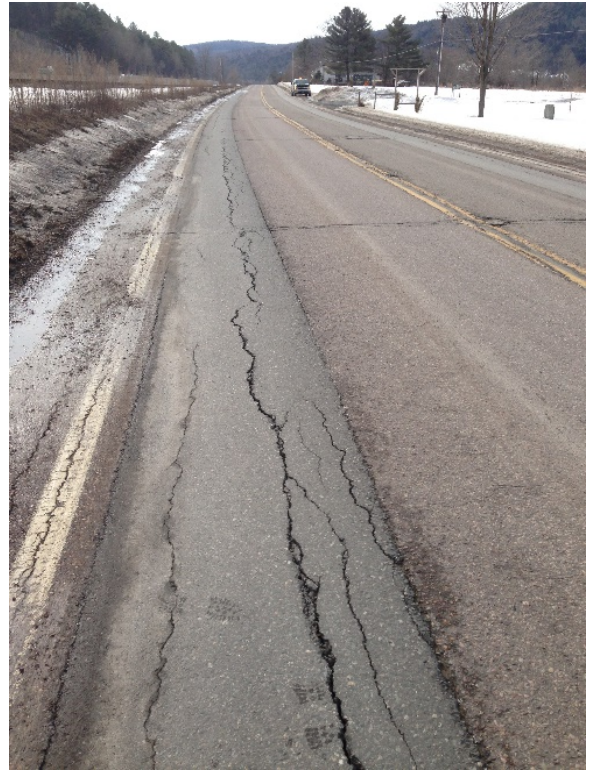
Test Site 2--Westbound
