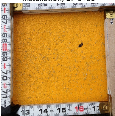
Recess Polyurea Wet Reflective, Installation, 17-0+00
