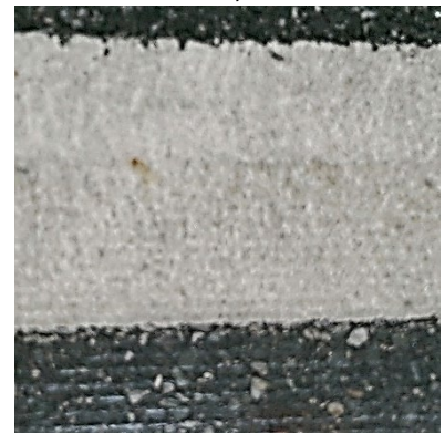
Recess Polyurea Wet Reflective, 36 months, 17-0+00
