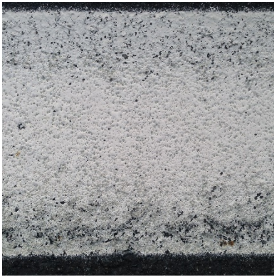
Surface MMA Utah, Installation, 11-0+00
