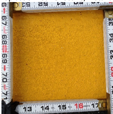
Recess Thermoplastic Wet Reflective, Installation, 23-0+00
