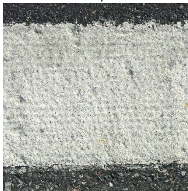
Recess Polyurea Utah, 15 months, 19-0+00
