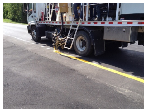
Figure 14: Optic package and paint being applied.
