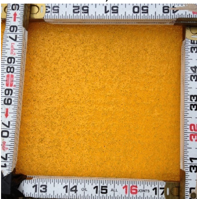
Recess Polyurea Utah, Installation, 19-0+00
