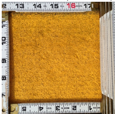
Recess Waterborne Paint, Installation, 4-0+00
