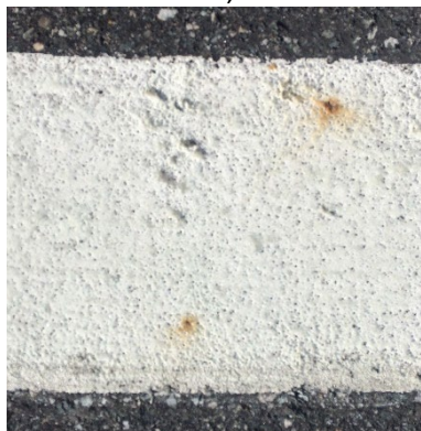
Recess Epoxy Utah, 15 months, 35-0+00
