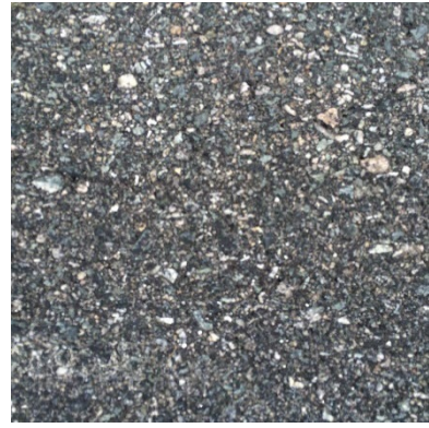
Surface Thermoplastic Wet Reflective, 8 months, 25-4+00
