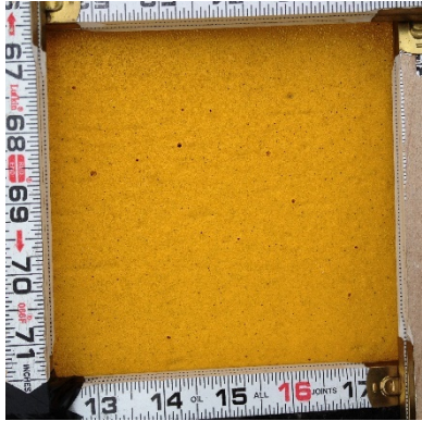
Recess Thermoplastic Utah, Installation, 22-0+00
