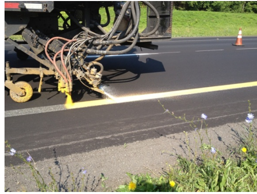
Figure 5: Waterborne binder and optic package being applied.
