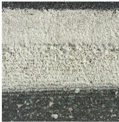
Recess Polyurea Wet Reflective, 15 months, 17-0+00
