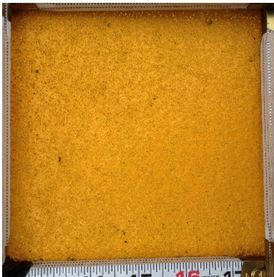
Surface Polyurea Utah, Installation, 13-0+00
