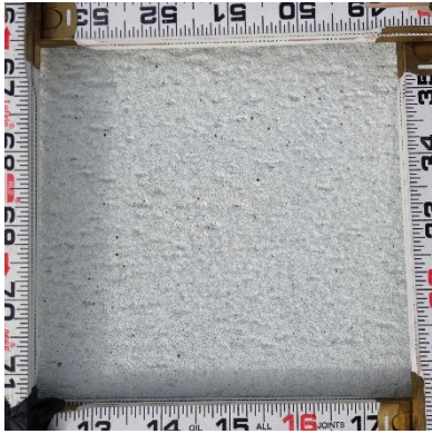
Surface Thermoplastic Utah, Installation, 28-1+00
