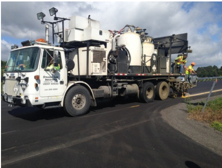
Figure 11: Epoxy markings being applied by the truck.
