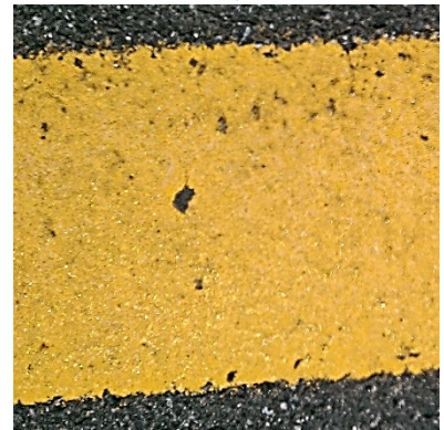
Surface Polyurea Utah, 36 months, 13-0+00
