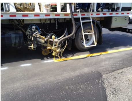
Figure 13: MMA markings being applied by the truck with double drops.
