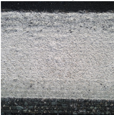
Recess MMA Wet Reflective, Installation, 7-0+00
