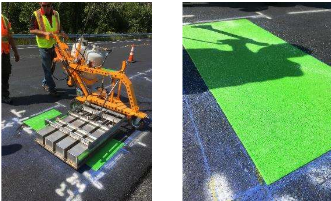
Figure 3: PreMark Installation
