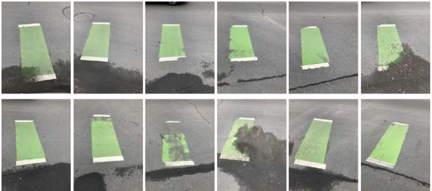
Figure 19: CycleGripMMAX Condition Location 2
