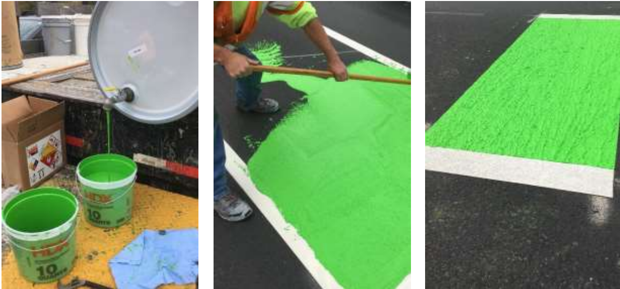
Figure 10: Color-Safe Installation
