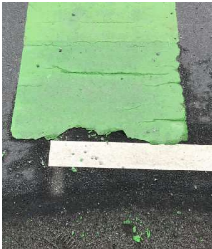
Figure 16: PreMark Delamination
