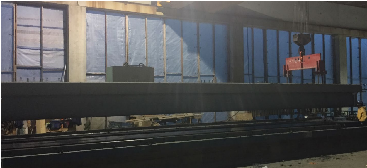
Figure 9.10: NEXT beam field testing of craned form removal
