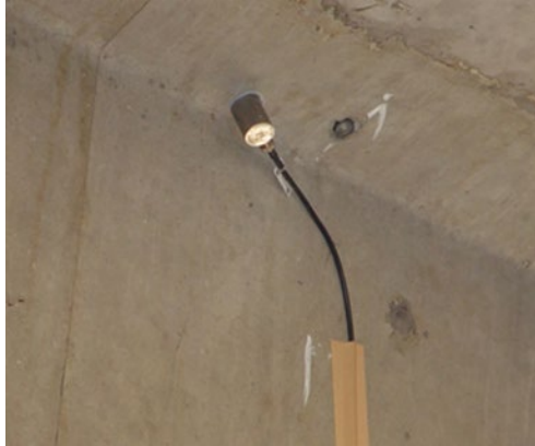
Figure 1.2: Acoustic emission sensor attached to a concrete girder (reference)
