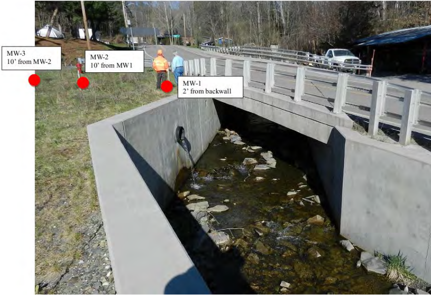
Figure 5.4: Williamstown piezometer installations
