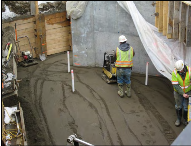
Figure 5.2: Bridgewater piezometer installation
