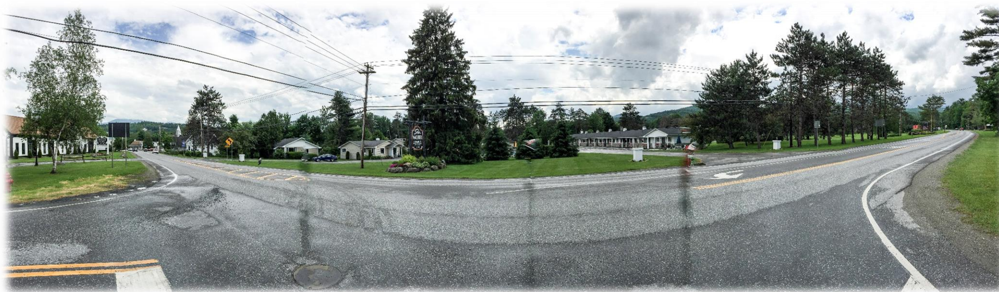
Mountain Road at Cottage Club Road
