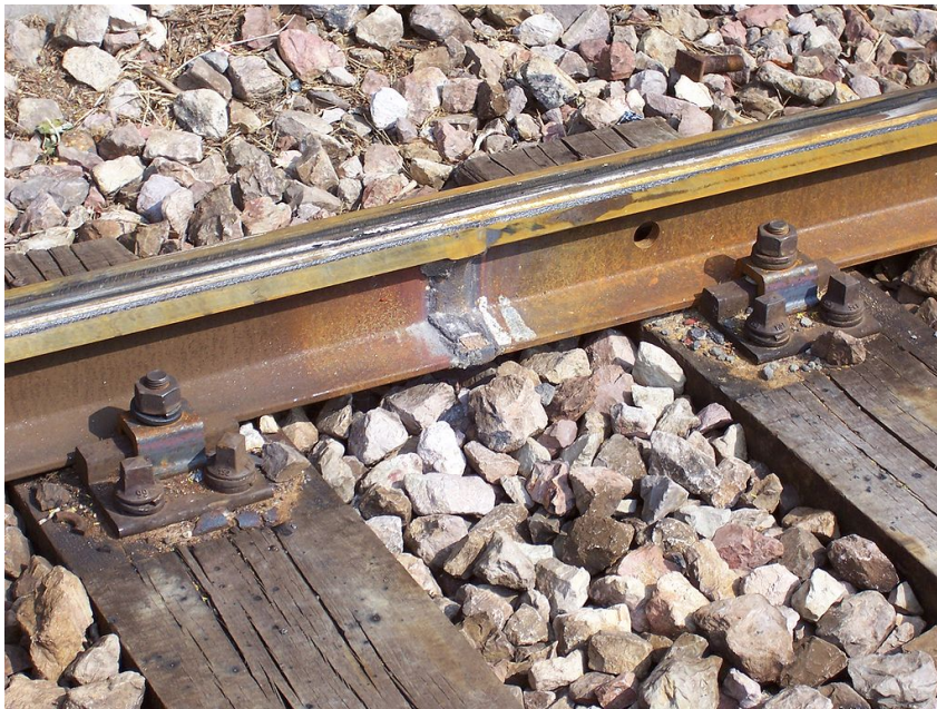
FIGURE 3.7 WELDED RAIL JOINT
