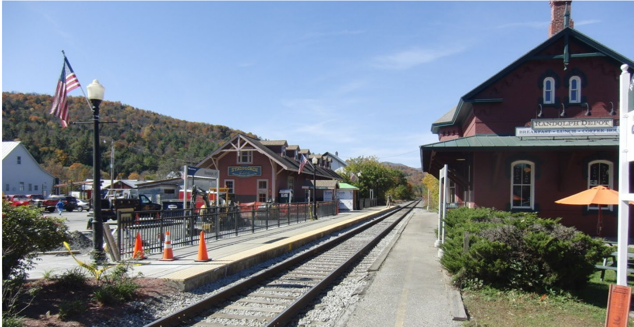
FIGURE 4.8 RANDOLPH STATION PLATFORM RENOVATIONS
