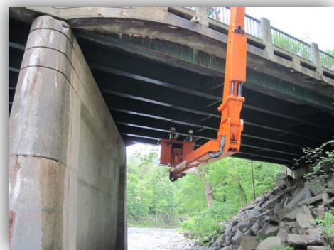
VTrans bridge inspectors at work.
