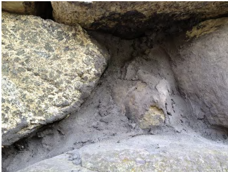
Figure 14 Up-close view of stone pointing and mortar work (VTrans 2013)
