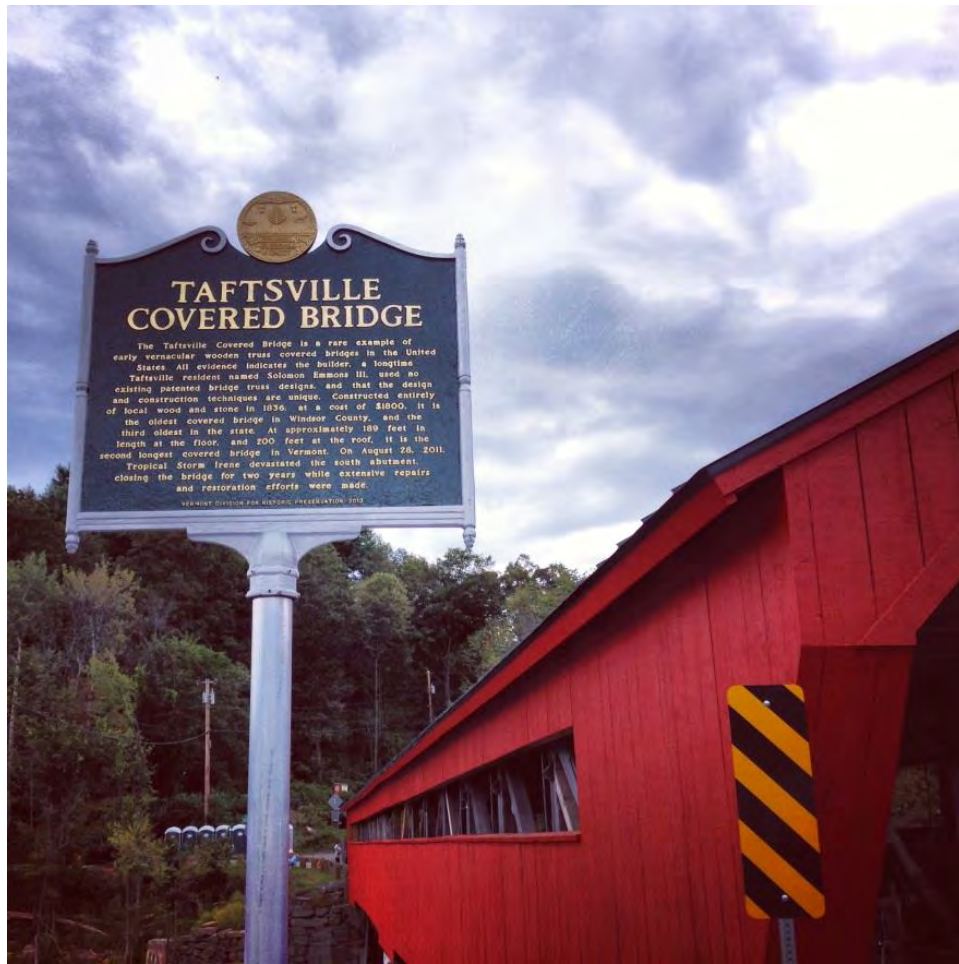
Figure 4 New historic plaque at the Taftsville Covered Bridge (VTrans 2013)
