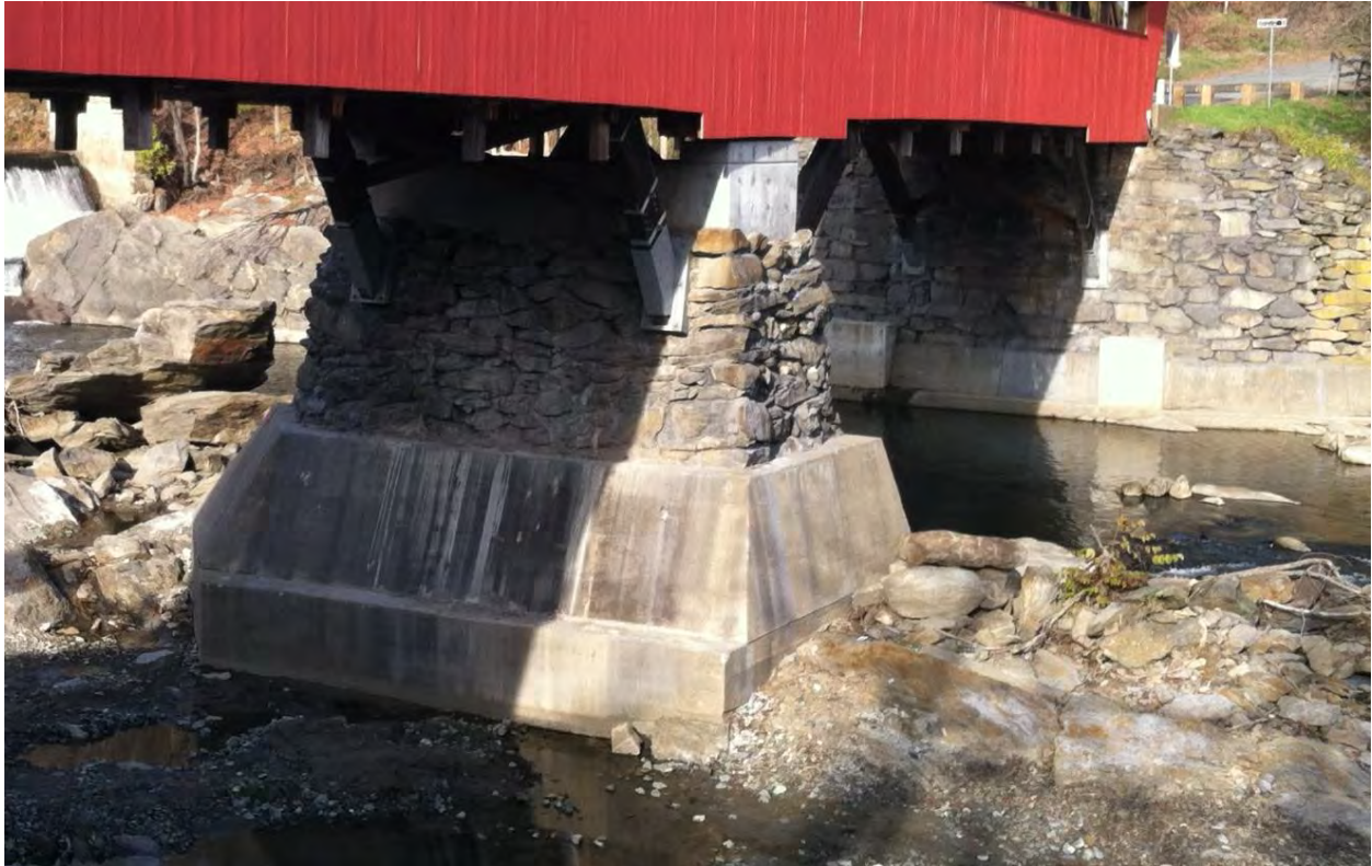
Figure 17 Completed pier showing the concrete cap and abutment (VTrans 2013)
