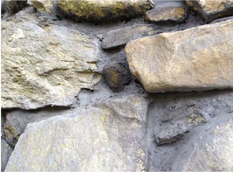
Figure 15 Completed mortar work (VTrans 2013)
