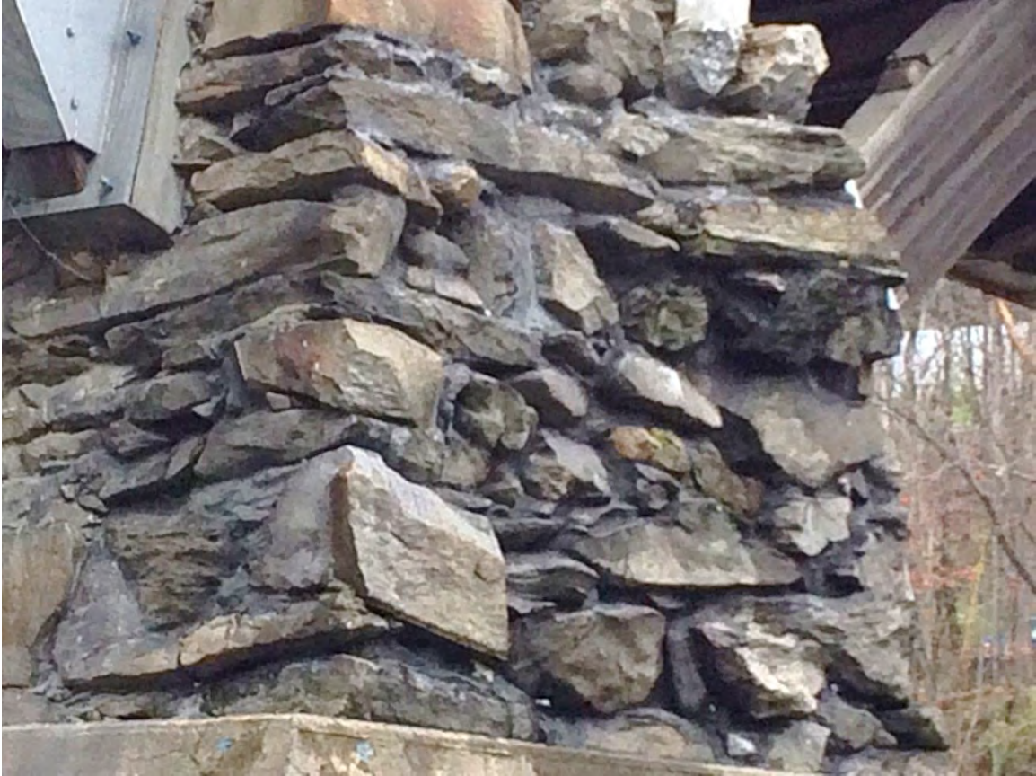
Figure 21 Downstream face of pier showing final construction (VTrans 2014)
