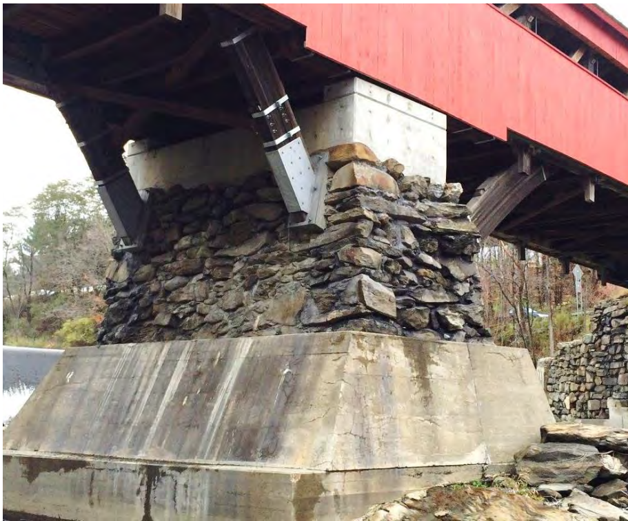
Figure 20 Pier after Construction in 2014
