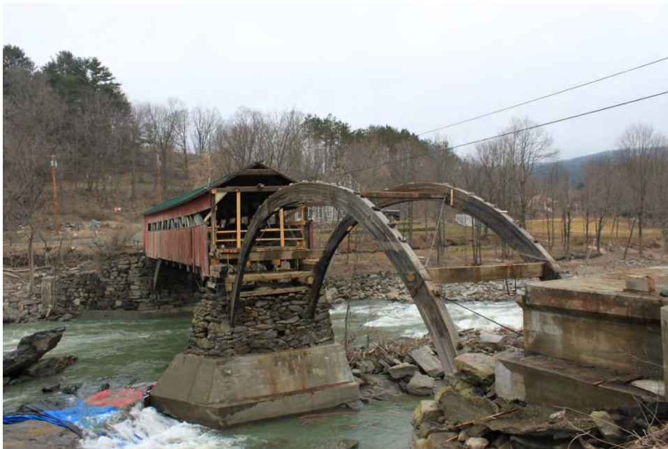
Figure 9 Westerly span dismantled leaving only the arches (VTrans, 2011)
