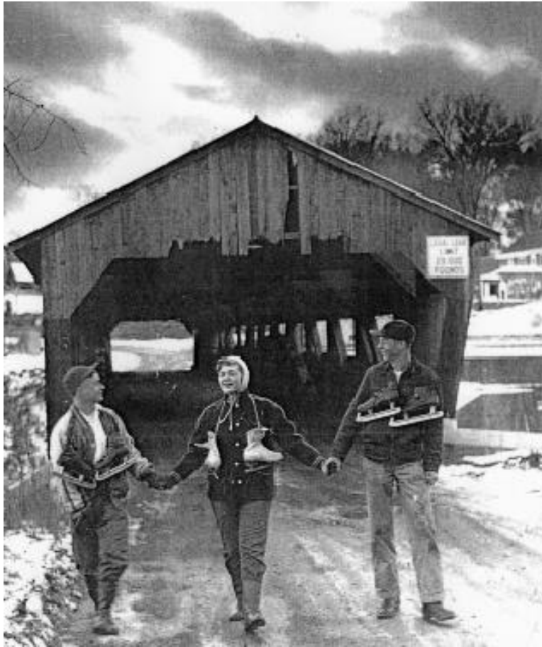
Figure 1 Taftsville Covered Bridge in the 1940's
