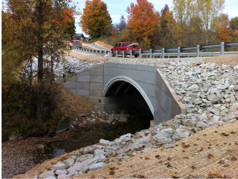
Figure 13 Completed Bridge in a Backpack (VTrans)
