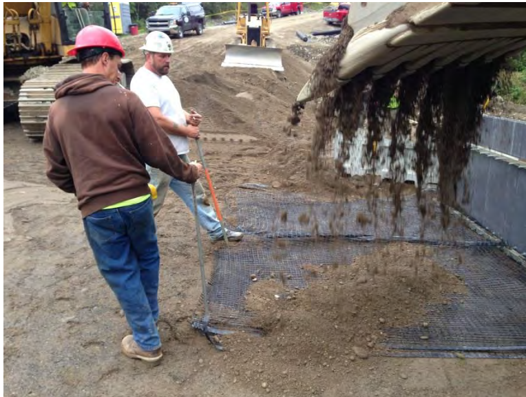
Figure 12 Applying subbase material over geotextile layers (ATI)
