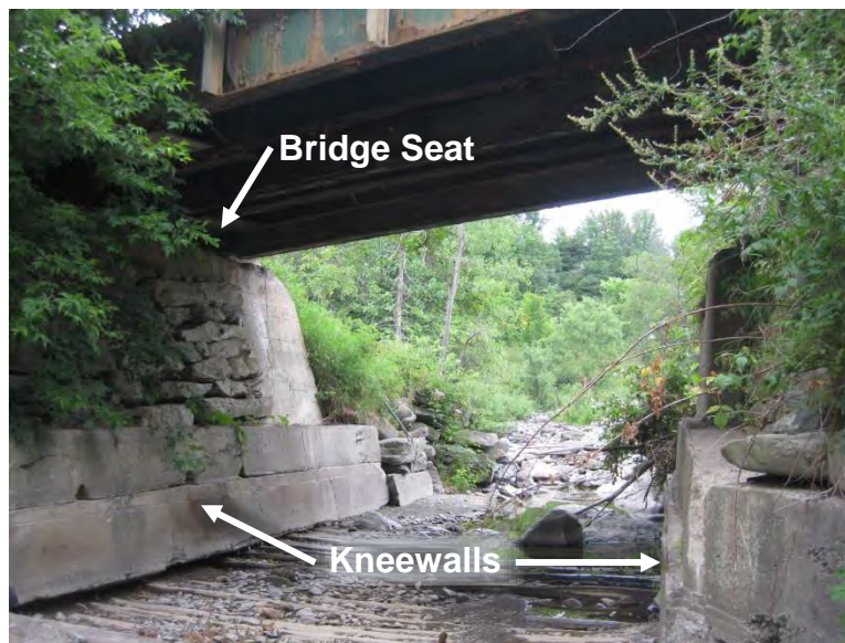
Figure 6 Existing substructure (VTrans)
