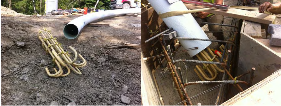
Figure 9 Anchorage reinforcement of the tubes (VTrans)
