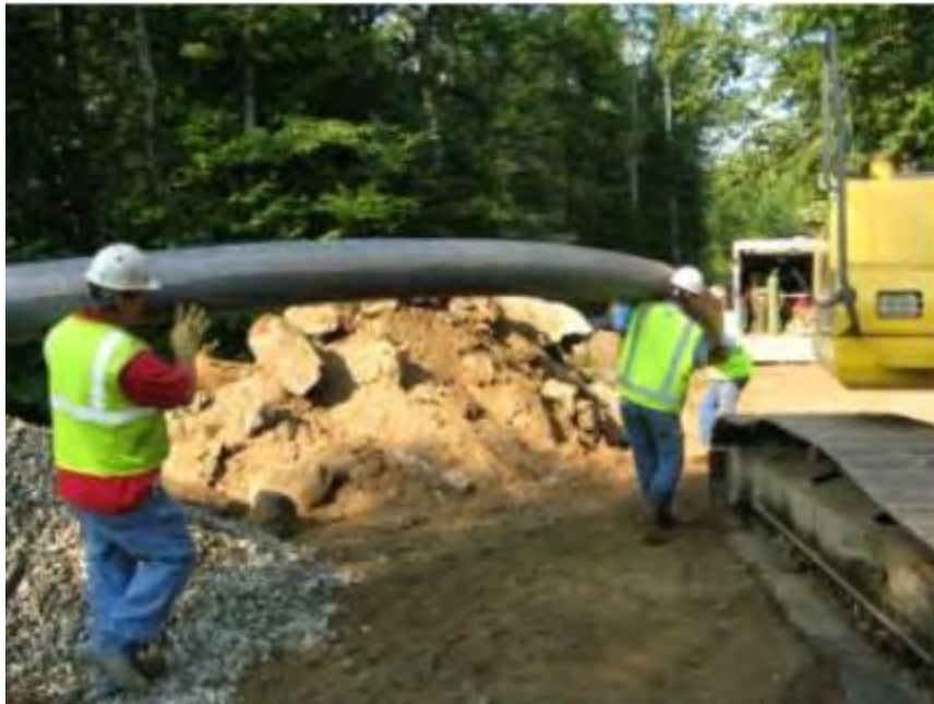
Figure 1 FRP tubes can be carried into place by hand labor. (AIT)
