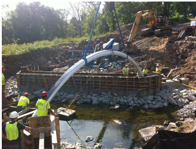
Figure 8 Installation of the first tube (VTrans)
