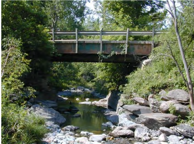
Figure 4 Bridge 48 profile (VTrans)
