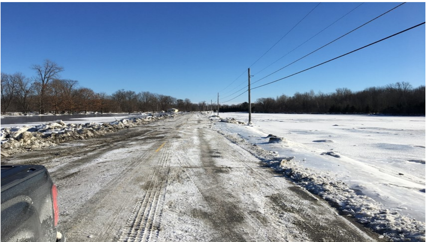
January - Route 78 Swanton, flooding cleanup
