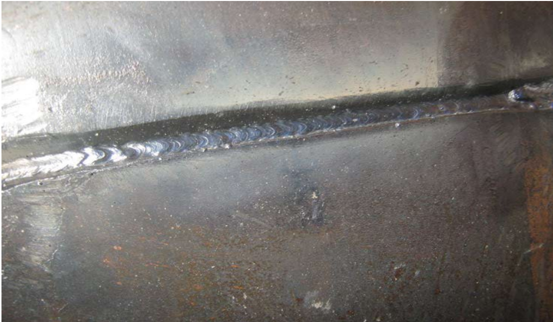
Root pass of a full penetration groove weld free of slag and ready for additional passes.
