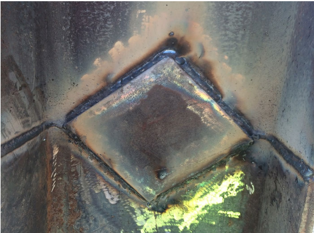
Completed backgouge and subsequent back side weld, as well as splice plate weld
