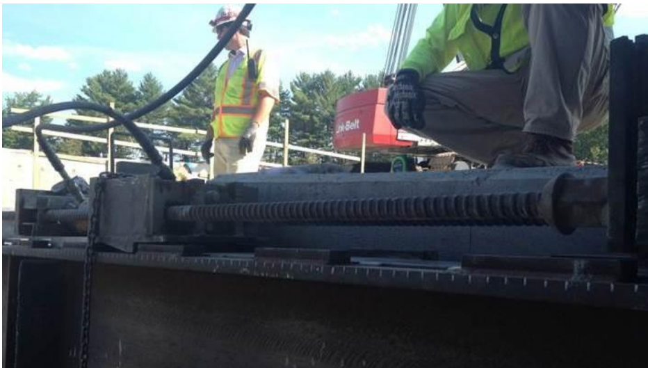
Southbound Slide System (Bridge pulled)
