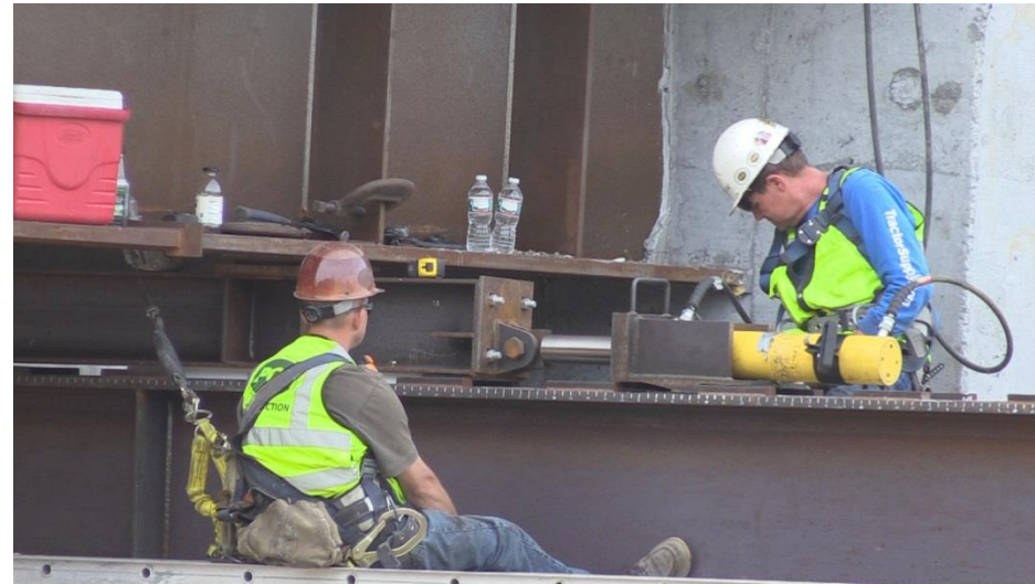
Northbound Slide System (Bridge Pushed)
