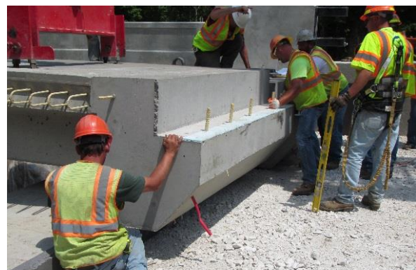
Figure 5: Precast Concrete Curtain Wall
