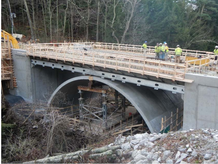
Figure 7: Bridge Elevation – Prior to Hanging Face Panels
