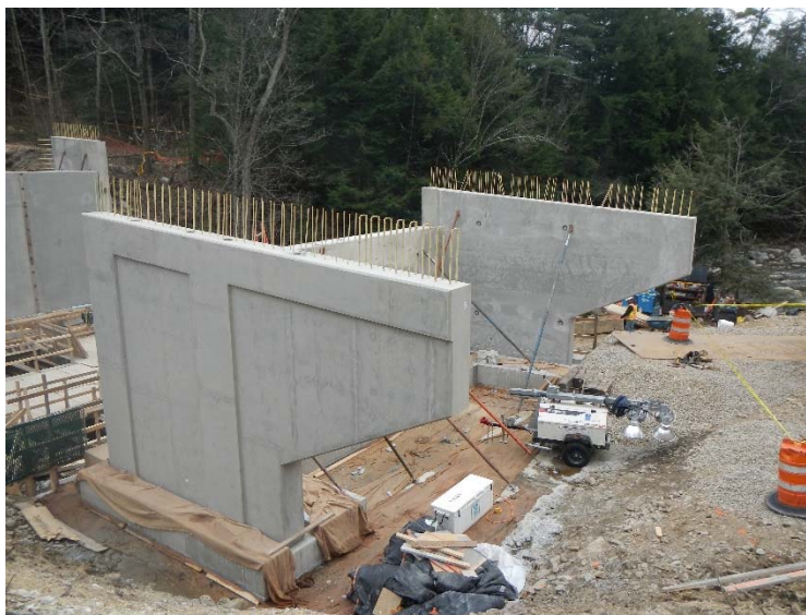
Figure 5: One Piece Precast Wingwalls 26' Long x 15' Tall
