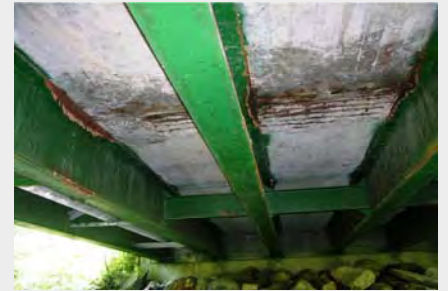
Deck Deterioration
