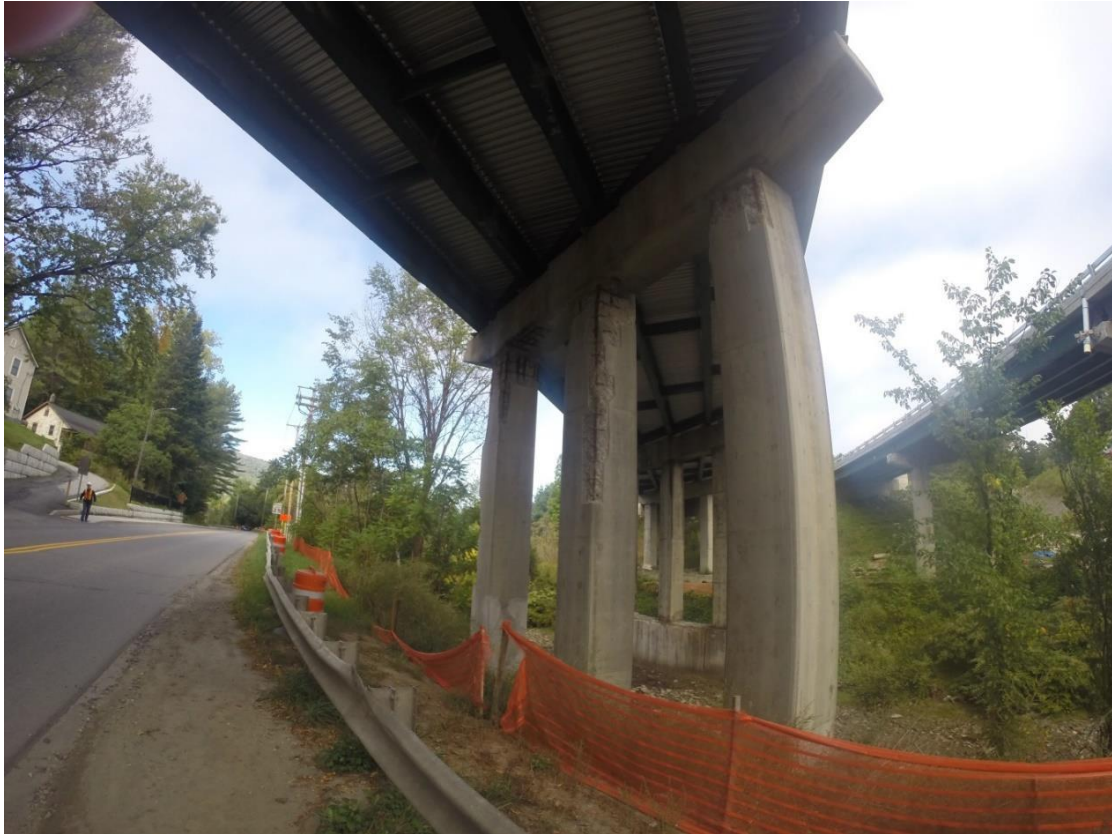
Figure 5.48 Pier on I-89 Waterbury Overpass Bridge with corners prepared for patch repairs
