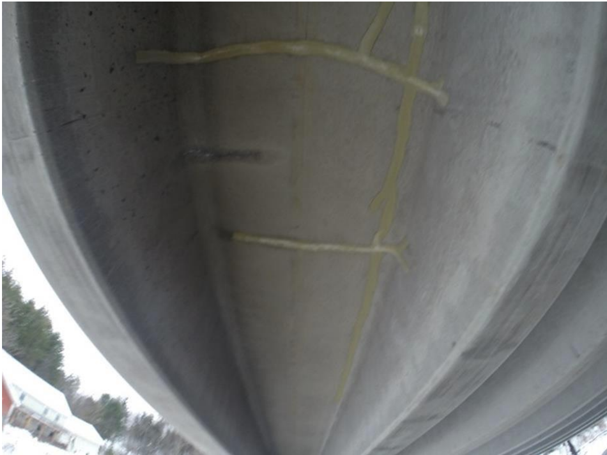
Figure 5.44 Girder cracks sealed Stowe Rte 100 Gold Brook Crossing Bridge
