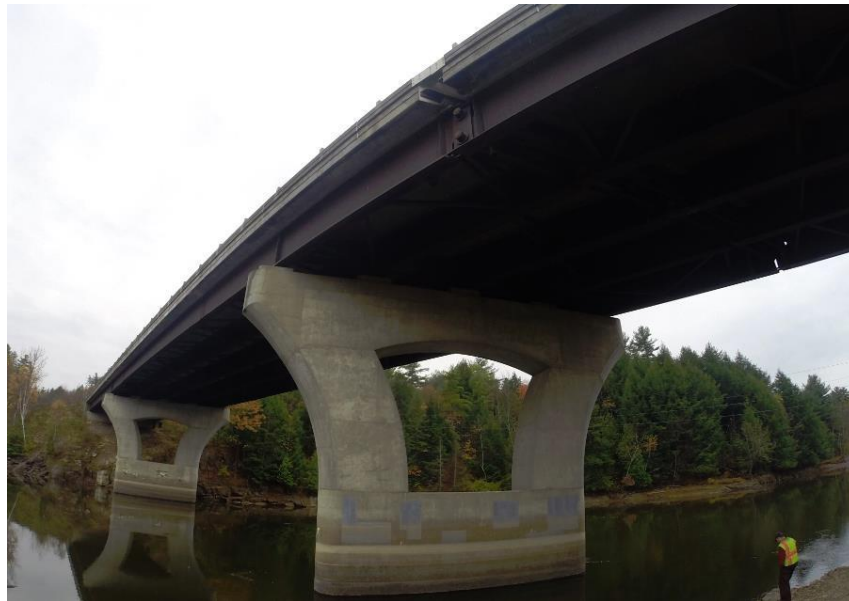
Figure 23: Bents, deck and beams
