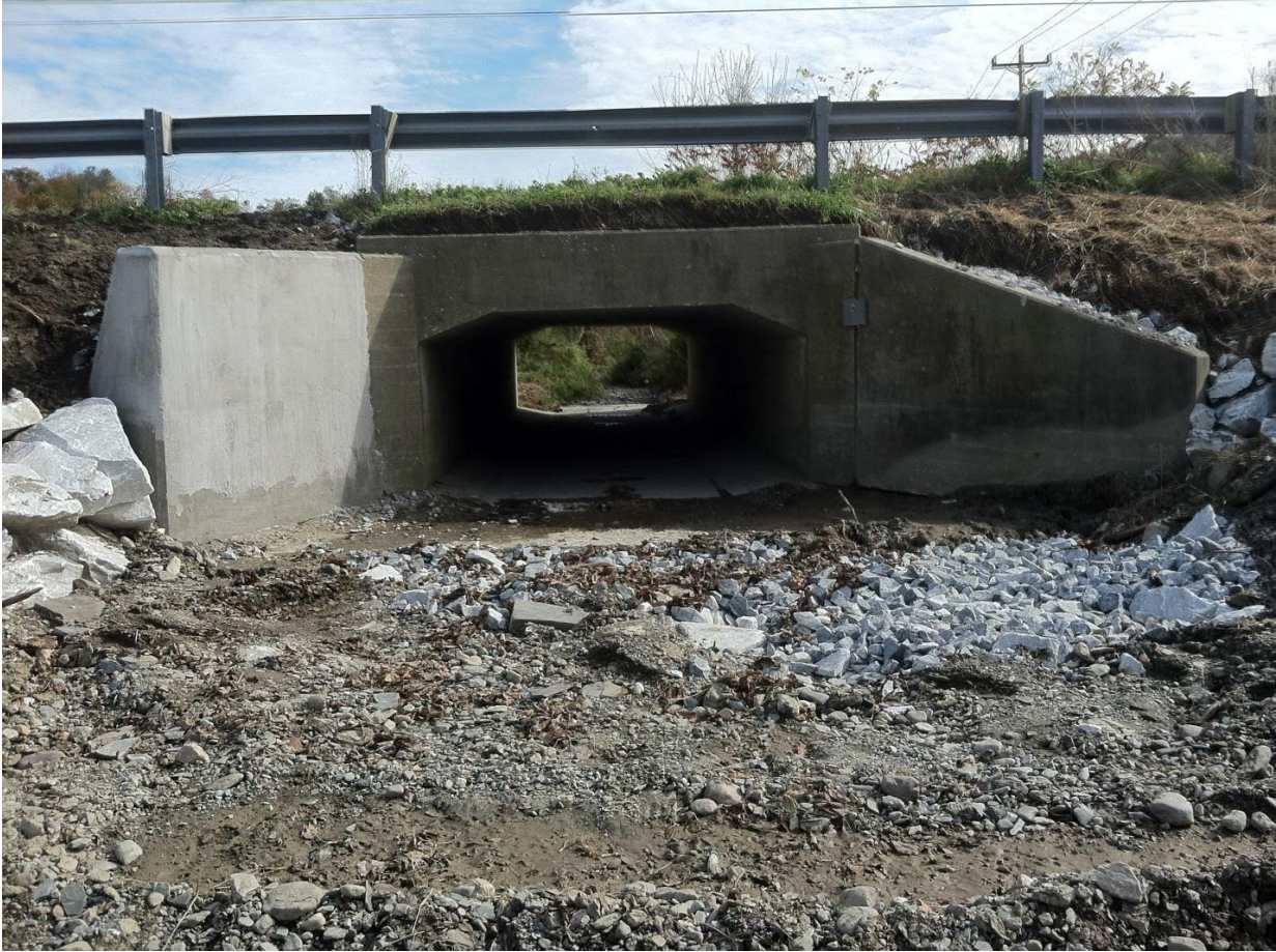
Figure 4.36 Vt. Rte. 30 Pawlet Br.#77 - REPAIRED Wing Wall/ Cut-off Wall Reconstruction $100,000
