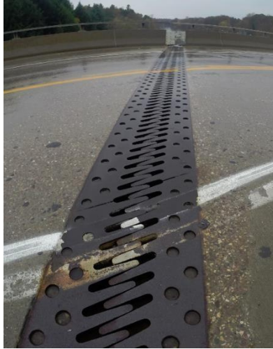
Figure 24: Steel finger joint. Notice no overlay on deck
