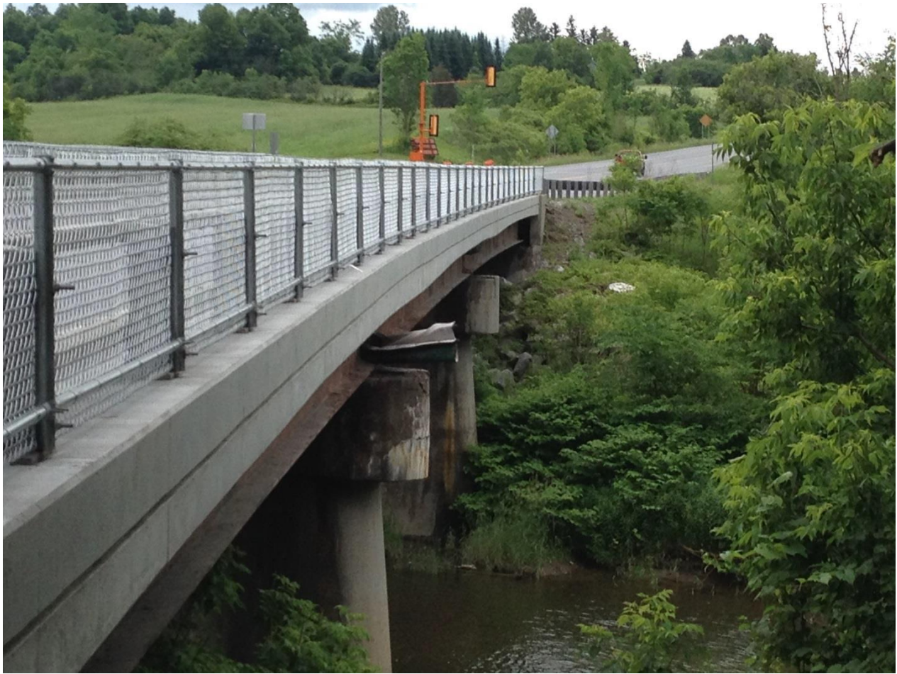
Figure 4.6 US 7 New Haven Br. #129 – REPAIRED Fascia/Curb Reconstruction, $350,000
