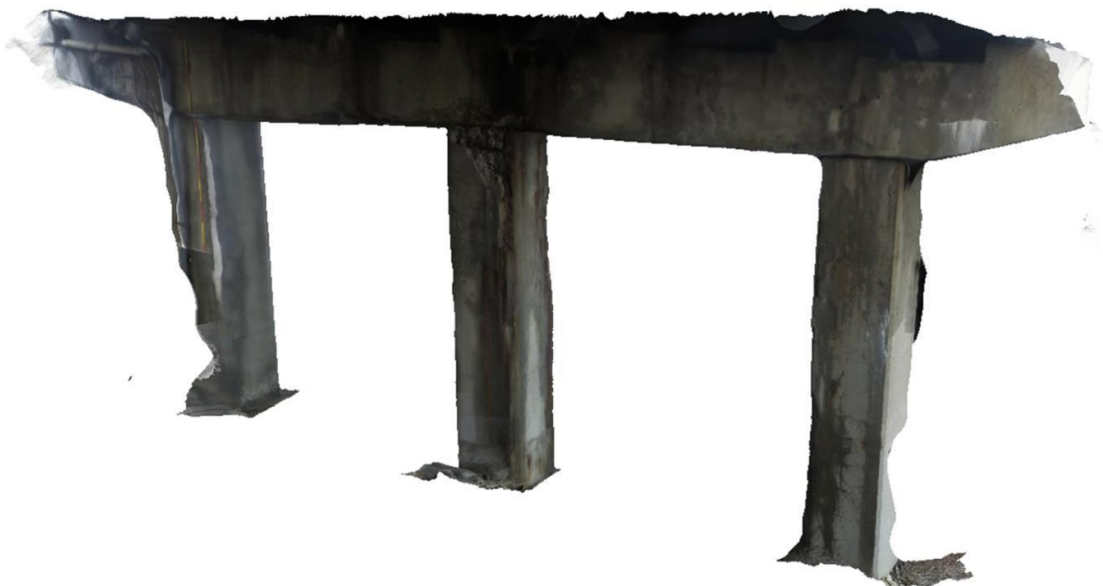
Figure 5.13 3-D photogrammetric point cloud rendering of Colchester/Milton I-89 Bridge
