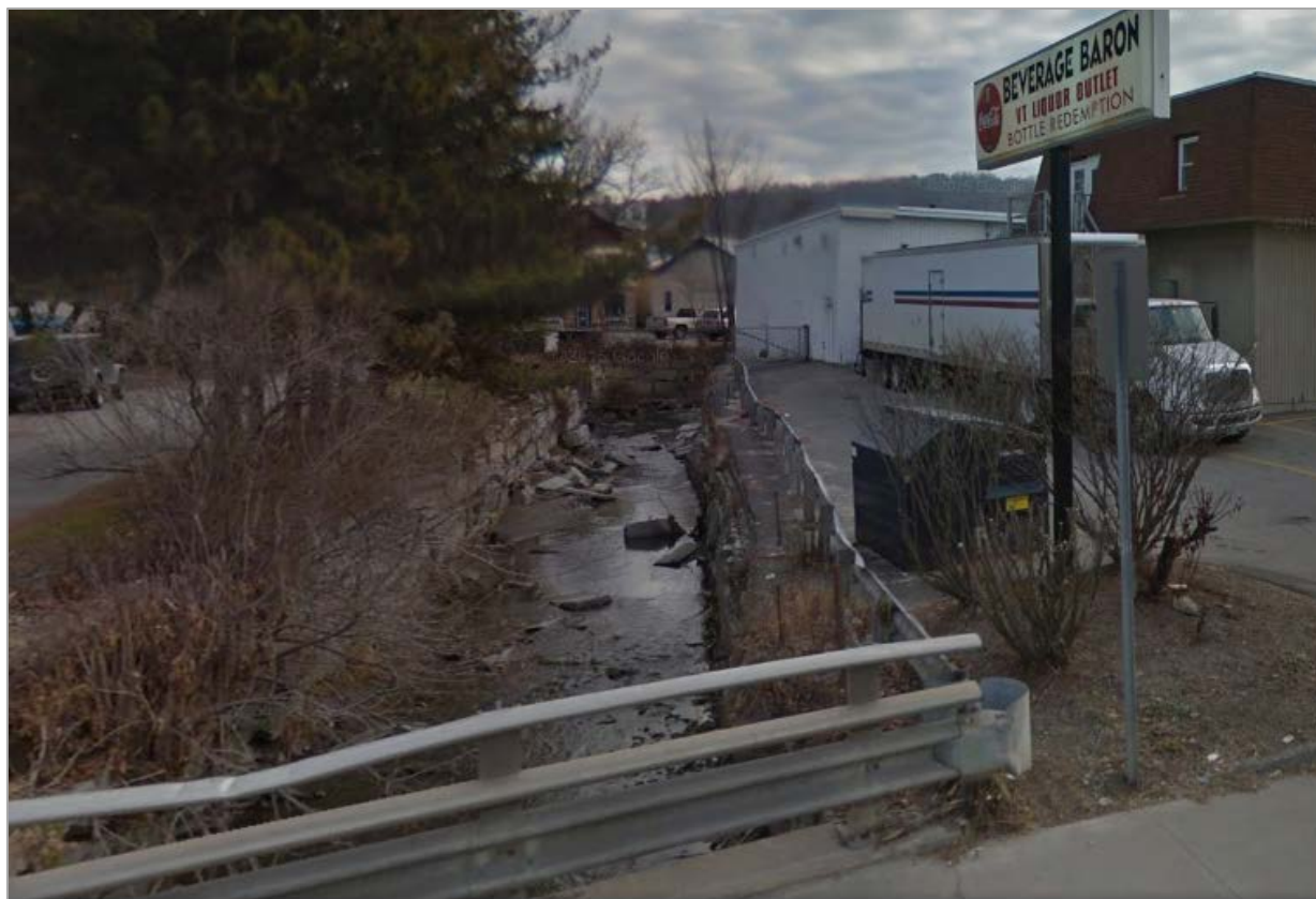
Figure 9 Armoring of Gunners Brook Upstream of U.S. Hwy 302
