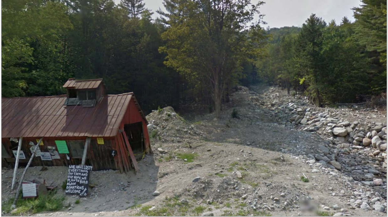
Figure 3 Money Brook Looking Upstream from Route 100 in Plymouth (August 2012)
