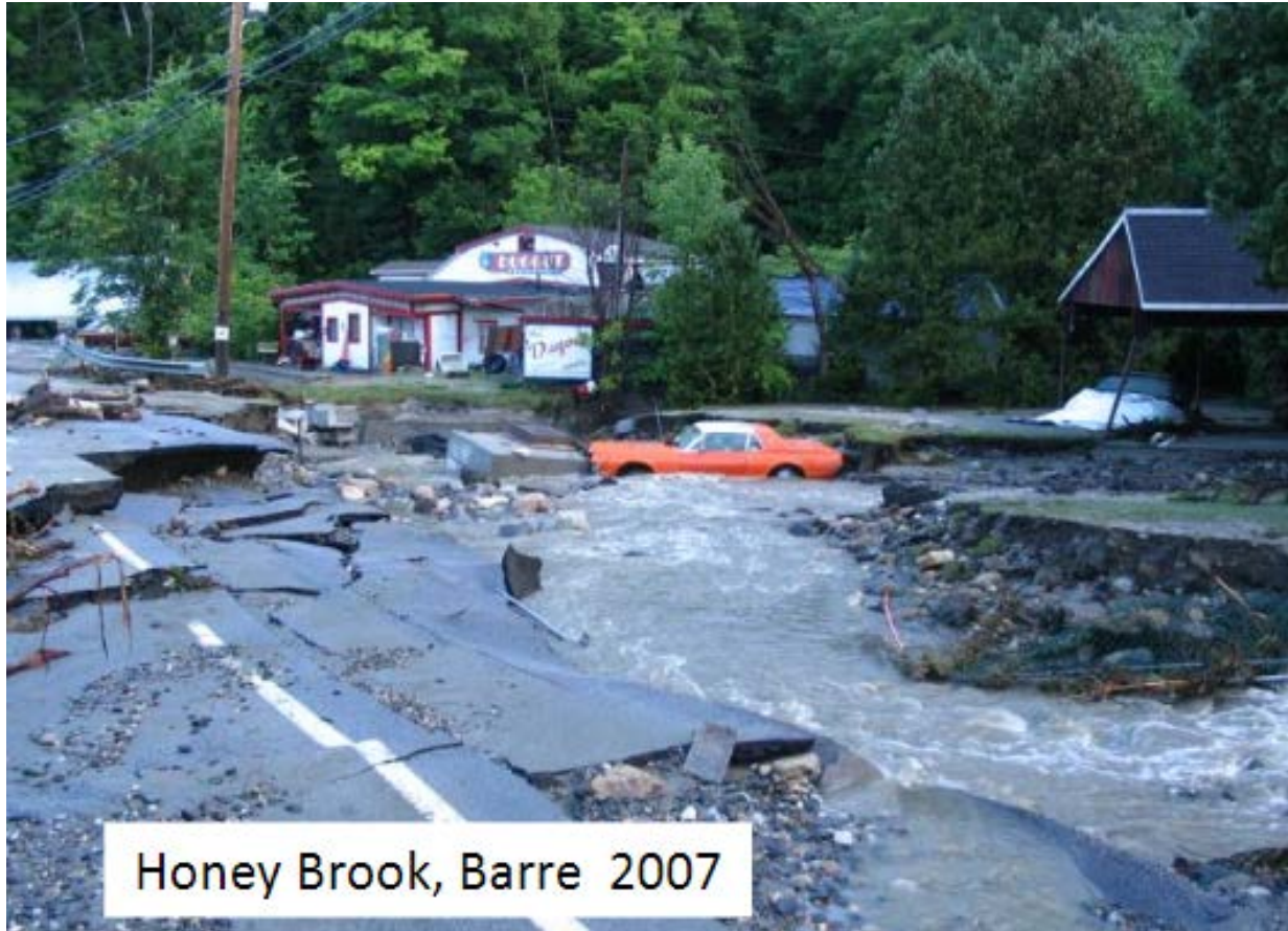
Figure 12 Flooding of Honey Brook at U.S. Hwy 302 in July 2007
