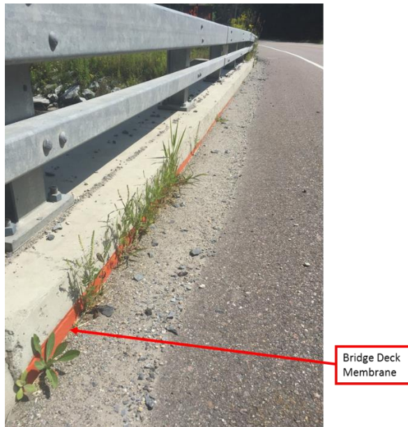
Figure 7: Bridge deck membrane
