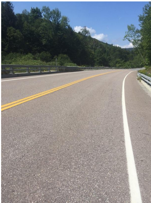
Figure 5: Bridge Overlay, looking north.
