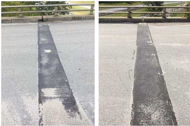
The photo on the left shows the bridge joint on the east end of the bridge while the photo on the right shows the bridge joint on the west end of the bridge. The bridge joints were in good condition.
