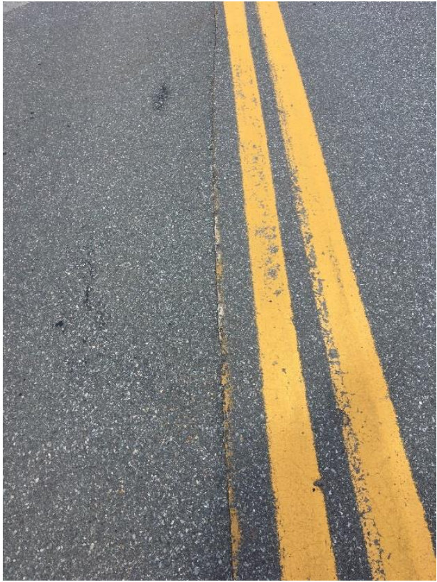
Close-up of the paving joint on Bridge 86.
