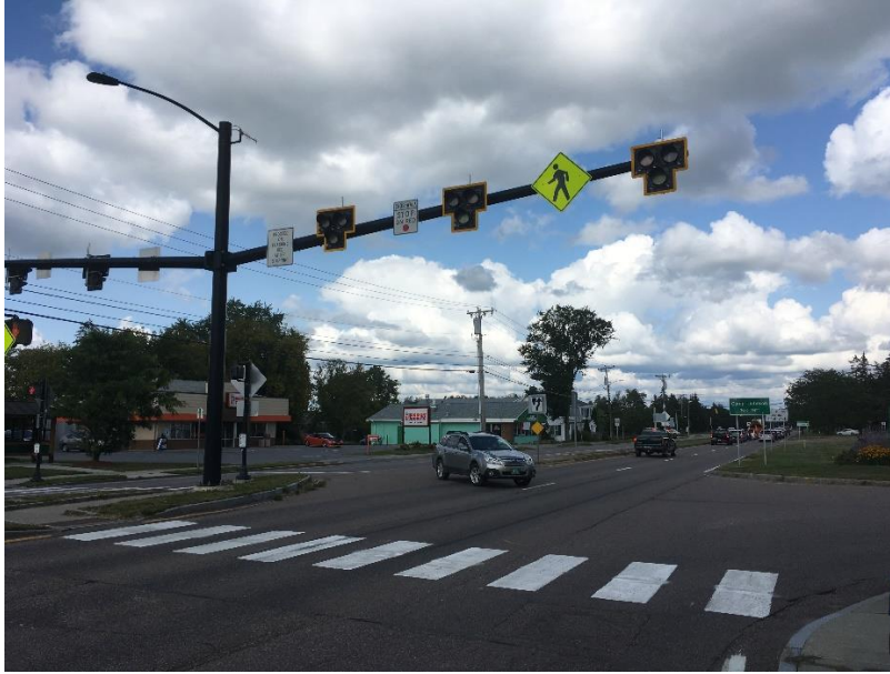
View of the HAWK Crosswalk System on the eastbound lane of VT Route 15 across from the Fanny Allen Hospital.
