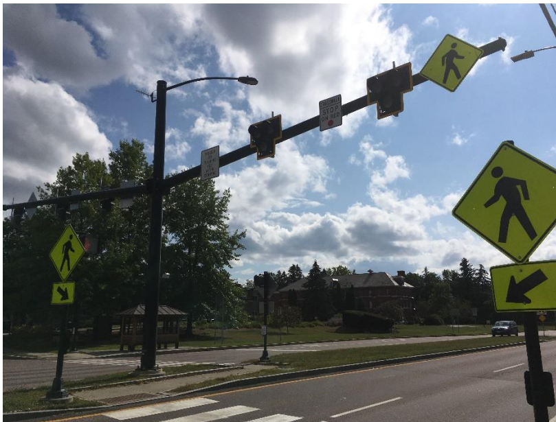
View of the HAWK Crosswalk System on the westbound lane of VT Route 15 across from the Fanny Allen Hospital.
