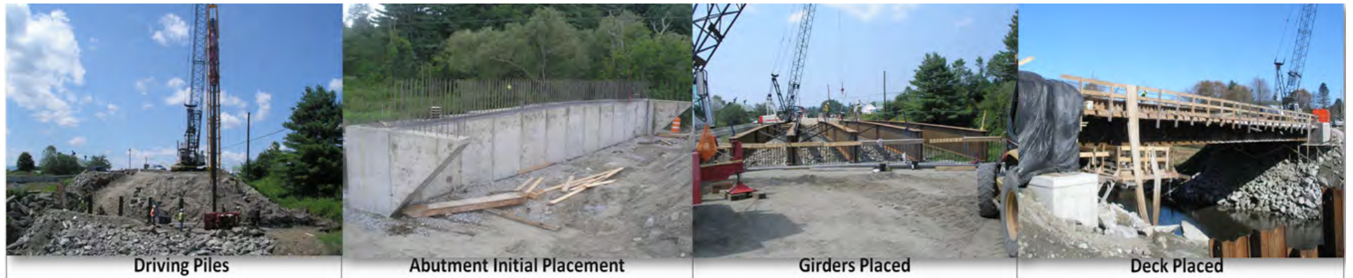
Figure C-5: East Montpelier Bridge Construction
