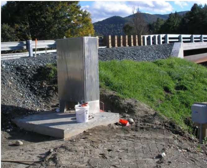
Figure 3-22: Data Acquisition System (Loggers) near Approach Slab
