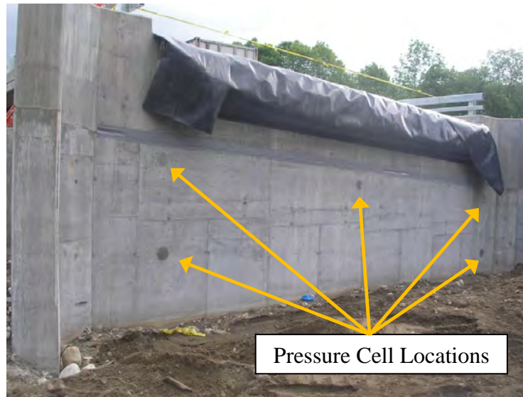
Figure 3-44: Abutment Pressure Cell during Backfilling at Stockbridge Bridge (Top Two Rows of Cells)
