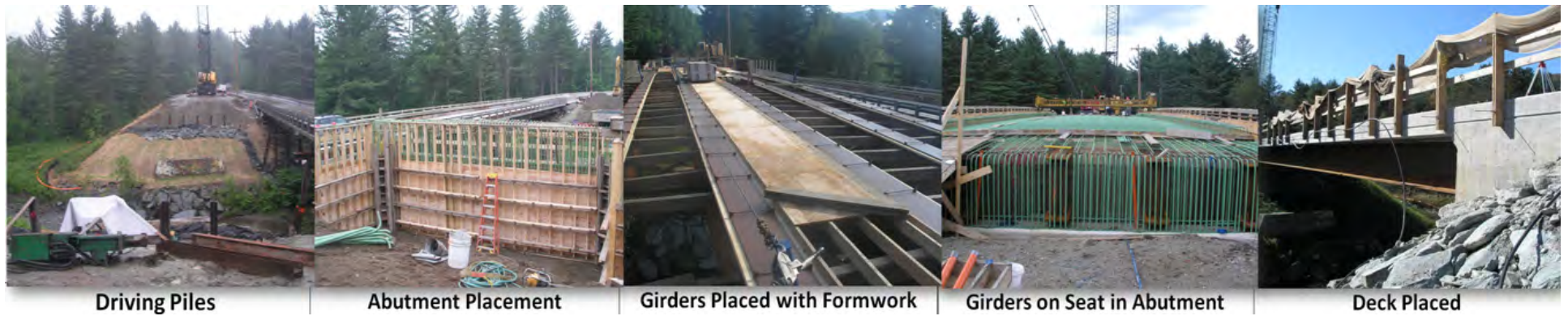
Figure C-4: Middlesex Bridge Construction
