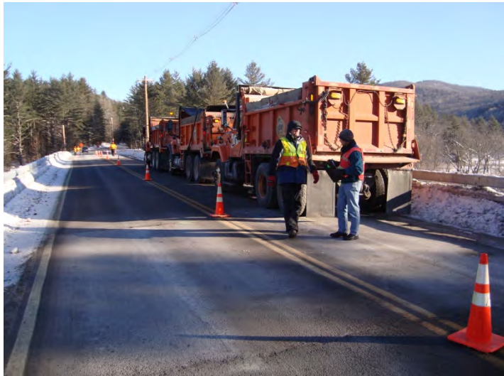
Figure 5-2: Middlesex Load Testing (Longitudinal Arrangement of Trucks)
