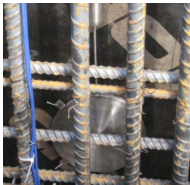
Figure 3-43: Earth Pressure Cell Installation
