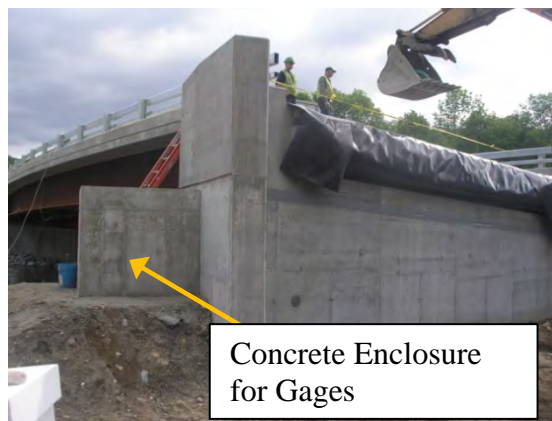
Figure 3-46: Displacement Transducer Enclosure
