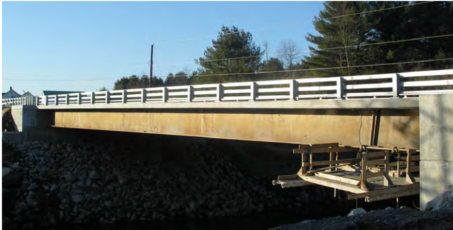
Figure 2-6: East Montpelier Bridge
