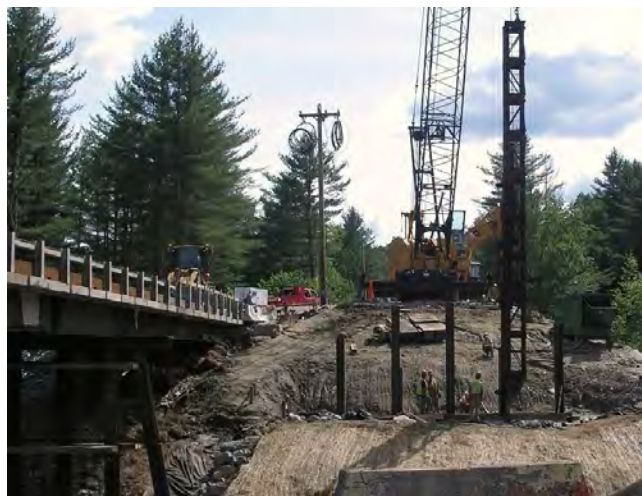
Figure 7-1: Pile Driving at the Middlesex Bridge
