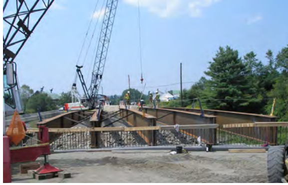
Figure 7-2: Girders Placed at the East Montpelier Bridge
