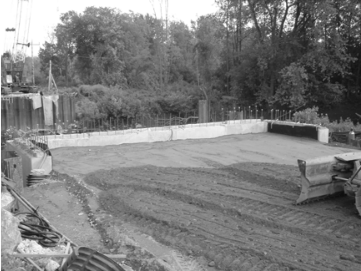
Figure 3.14 Placement of Granular Backfill.
