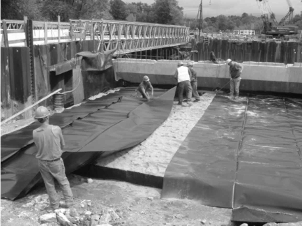
Figure 3.13 Installation of Flexible PVC Geomembrane.
