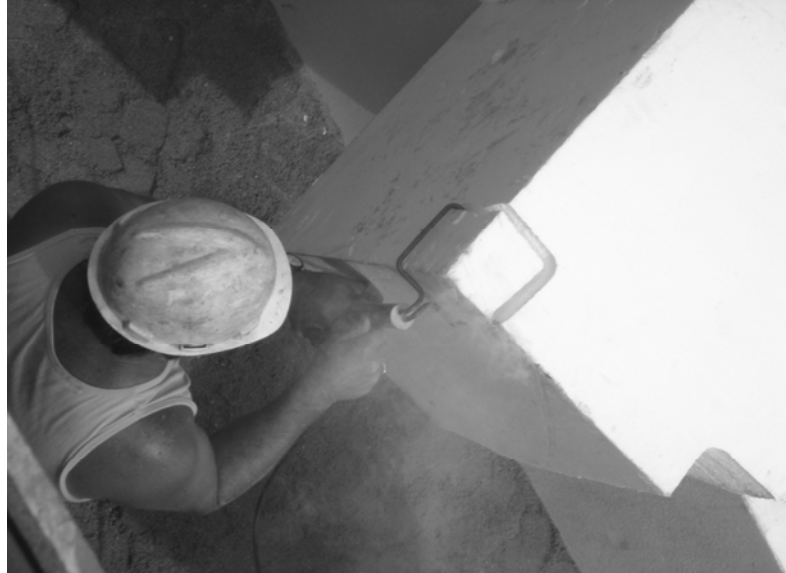
Figure 3.8 Trimming a GeoFoam Block.
