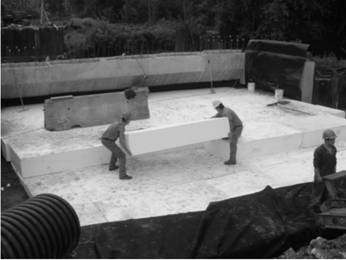
Figure 3.11 Placement of GeoFoam Blocks in Stepped Layers.
