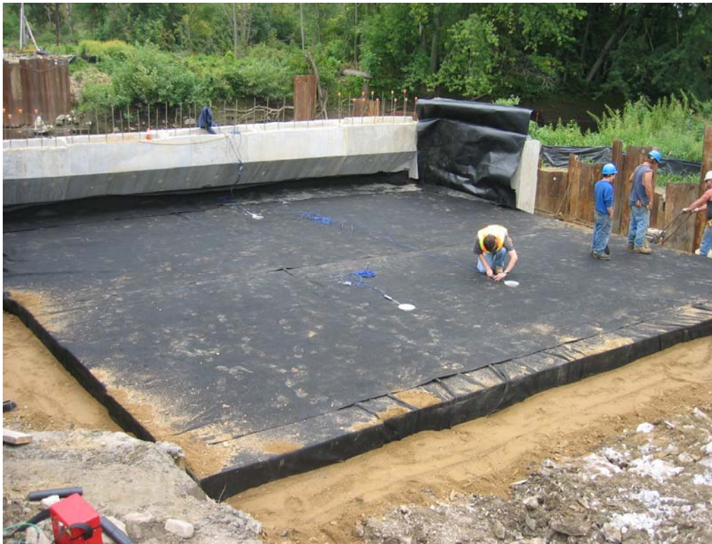
Figure 5.5. Installation of Earth Pressure Cells 1A4, 1A5, 1A6, 2A4, 2A5, 2A6.
