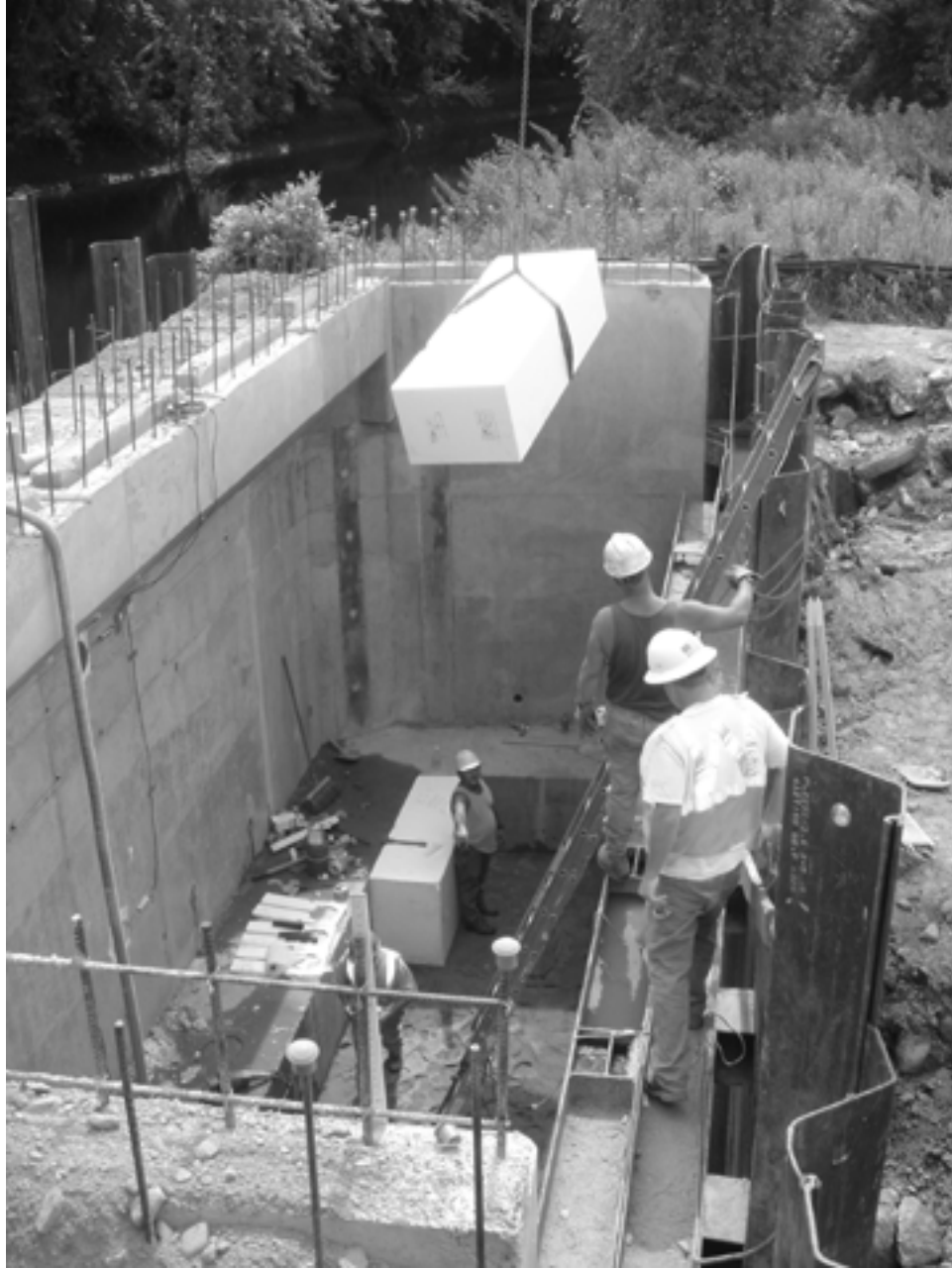
Figure 3.9 Placement of GeoFoam Blocks Adjacent to Abutment Footing.
