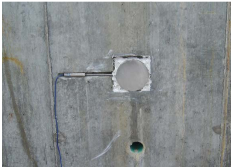
Figure 5.4. Installation of Earth Pressure Cells 1A2, 1A3, 2A2, and 2A3.
