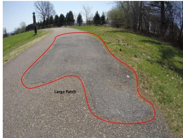
Figure 53 Test Spot with Large Asphalt Patch
