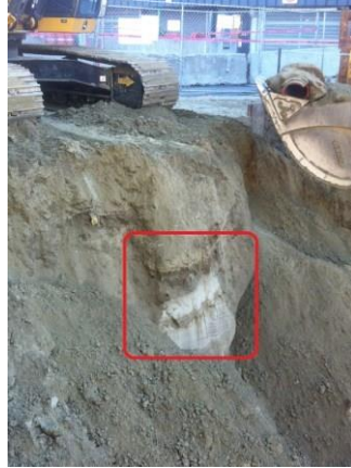
Figure 42 A layer is observed which is consistent with the GPR result in Figure 35
