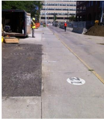
Figure 31 Test Site at St. Paul Street
