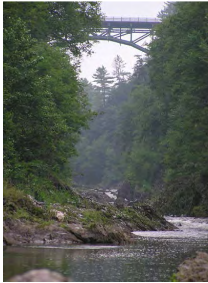
FIGURE 16 View of bridge from the Ottauquechee River (8).
