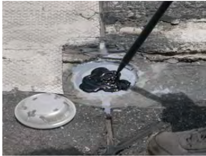
FIGURE 6 Epoxy application.
