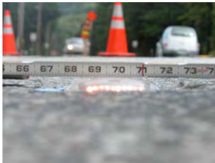
FIGURE 7 Domes are slightly above road surface.
