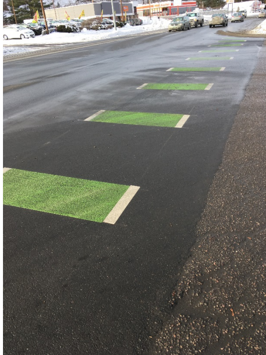
Figure 3: Big Lots Intersection Ennis-Flint CycleGrip MMAX Bike Lane
