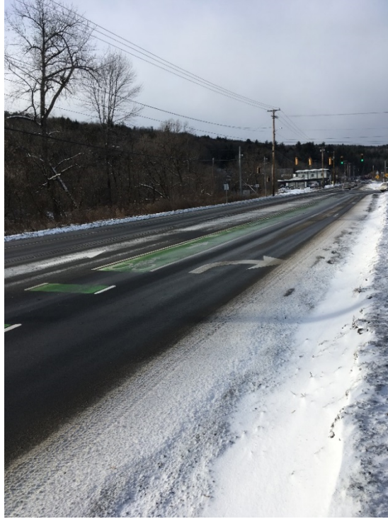
Figure 2: Price Chopper Intersection Ennis-Flint Thermoplastic Premark Bike Lane and Symbols
