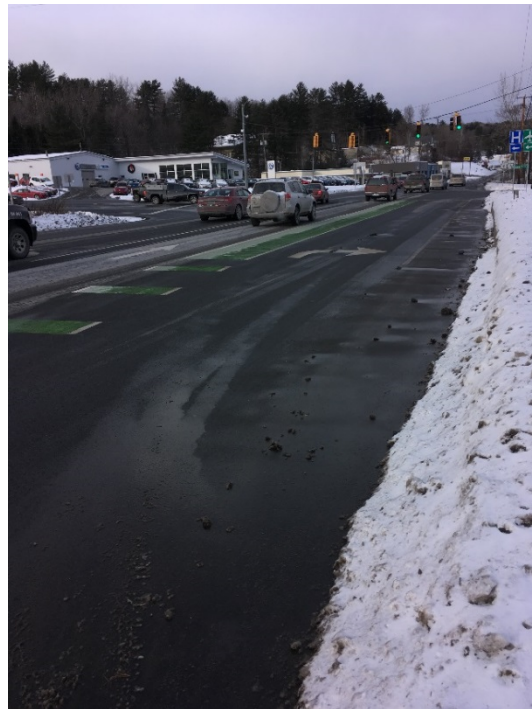
Figure 4: CVS Intersection Transpo Colorsafe Bike Lane and Brite-Line HDX Symbols
