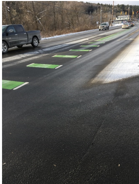
Figure 1: Price Chopper Intersection Ennis-Flint Thermoplastic Premark Bike Lane and Symbols
