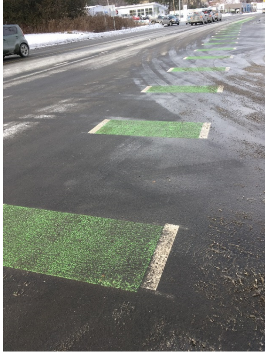
Figure 5: CVS Intersection Transpo Colorsafe Bike Lane and Brite-Line HDX Skips
