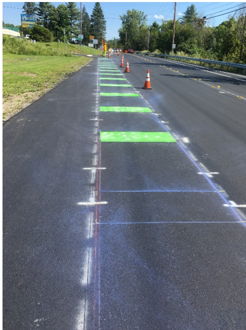
Figure 4: Installed PreMark Bike Lane Green Blocks
