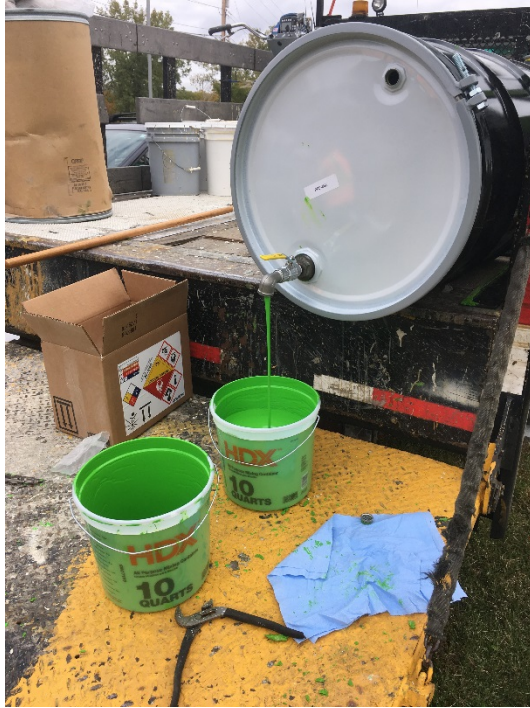
Figure 28: Pouring Methyl Methacrylate from Drum to make 2 Gallon Mixes
