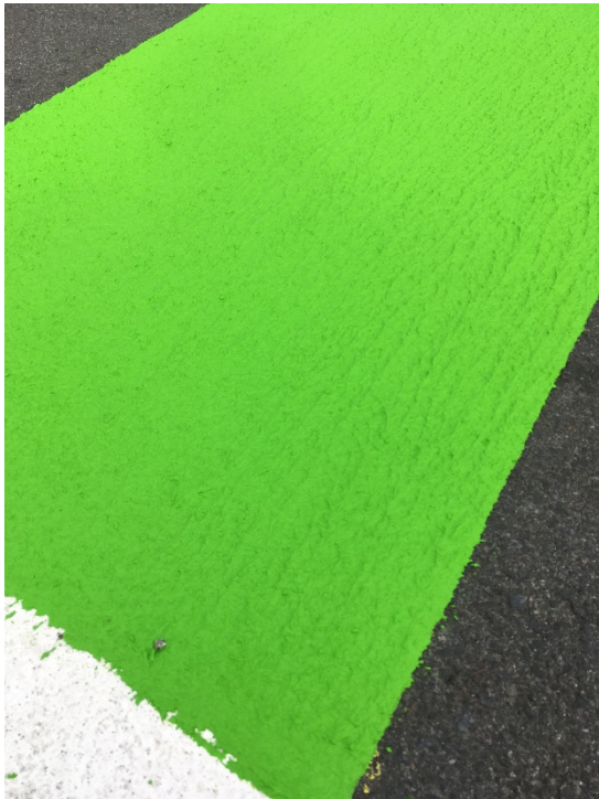
Figure 20: Close-up of CycleGrip MMAX at McDonald's Intersection
