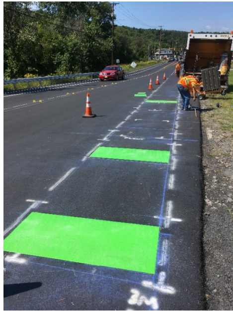
Figure 3: Laying out PreMark Bike Lane Green Blocks
