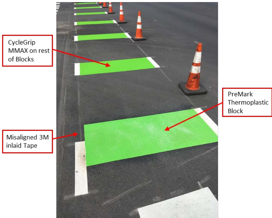
Figure 25: Eastbound side Bike Lane at McDonald's Intersection with both CycleGrip MMAX and PreMark Thermoplastic
