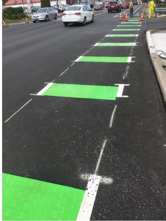
Figure 23: Applied PreMark Thermoplastic at McDonald's Section
