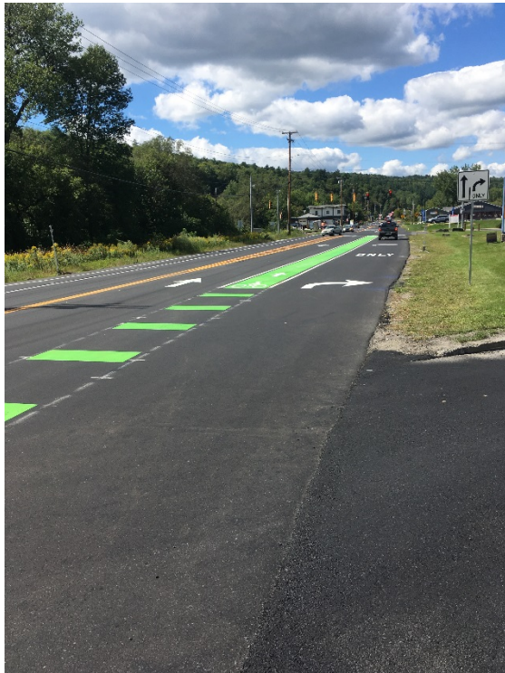
Figure 10: Completed PreMark Bike Lane at Price Chopper Intersection
