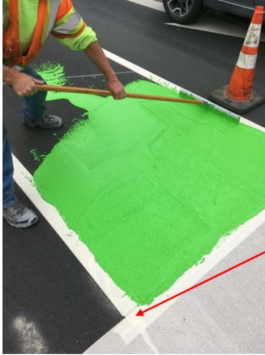
Figure 30: Application of Transpo Color-Safe at CVS intersection
