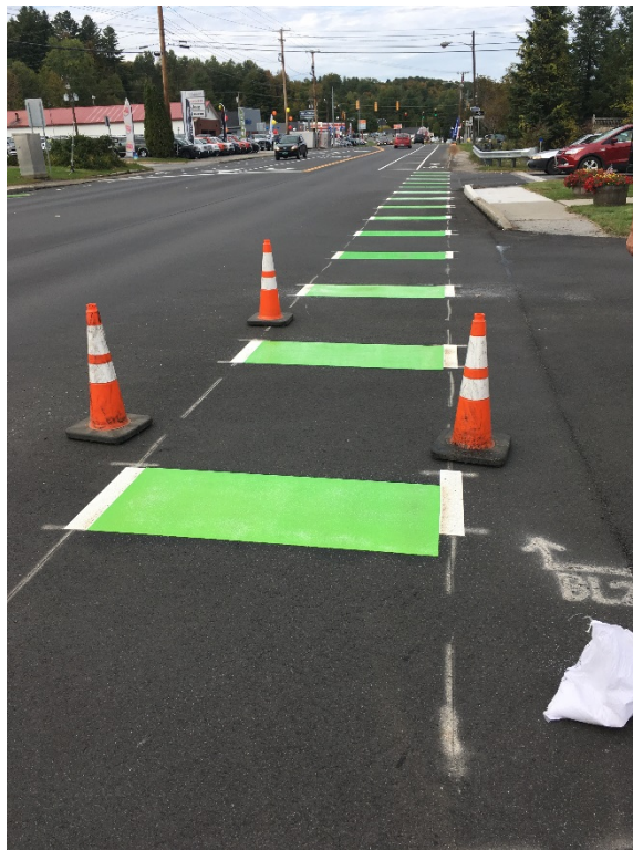
Figure 24: Completed Bike Lane Section at McDonald's Intersection
