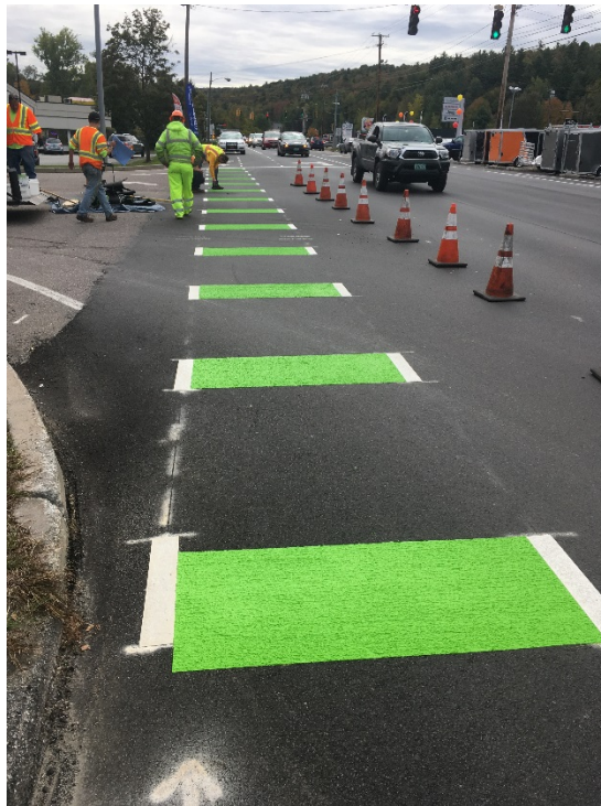
Figure 18: Finished CycleGrip MMAX section at the Vermont Shopping Center Intersection
