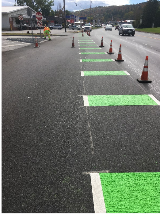
Figure 36: Finished Color-Safe Blocks Near CVS Intersection
