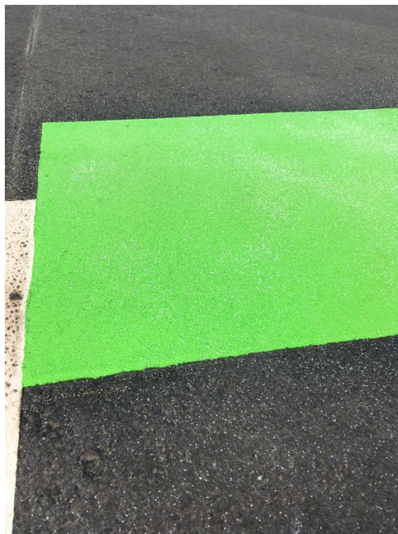
Figure 26: Close-up of PreMark Thermoplastic on Eastbound side at McDonald's Intersection
