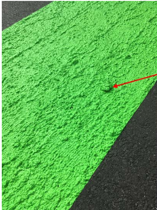
Figure 37: Close-up of Color-Safe Bike Lane Block with an Aggregate Clump
