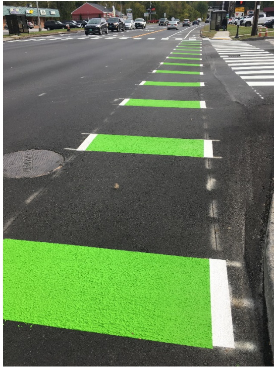
Figure 19: CycleGrip MMAX applied at McDonald's Intersection on the eastbound side. First 12 blocks.
