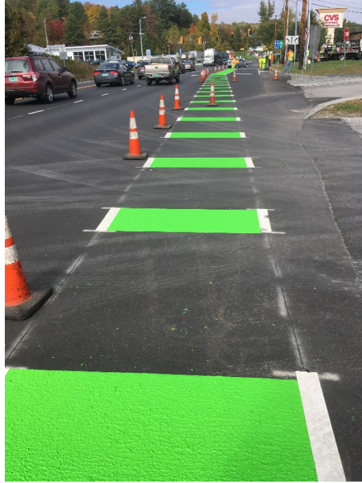
Figure 38: Finished Color-Safe Bike Lane Near CVS Intersection
