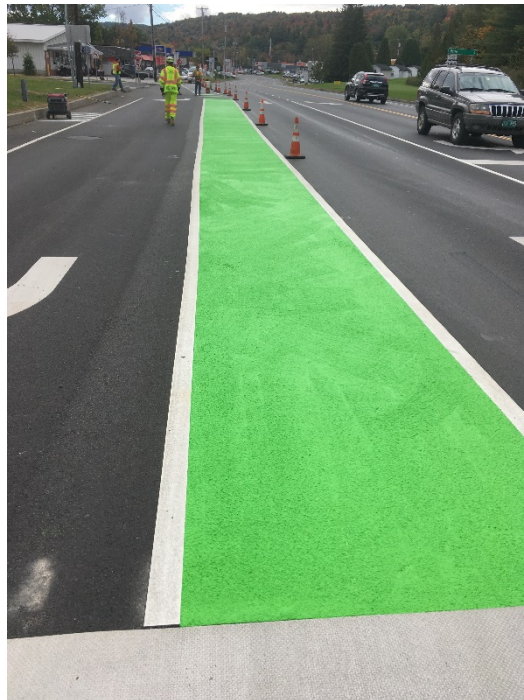
Figure 33: Finished Solid Section of Transpo Color-Safe at CVS intersection
