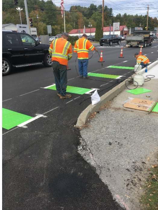
Figure 21: PreMark Thermoplastic applied at McDonald's Intersection on the westbound side
