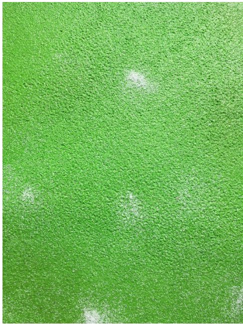
Figure 6: Close-up of Installed PreMark Bike Lane Green with anti-skid Corundum
