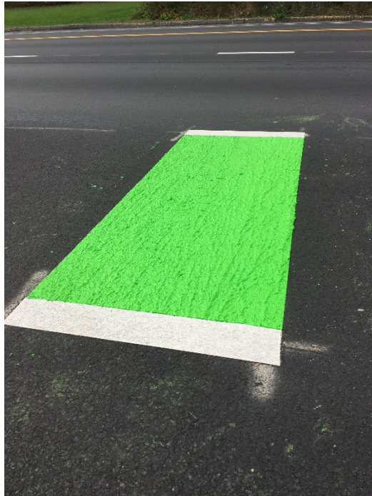
Figure 35: Finished Color-Safer Bike Lane Block
