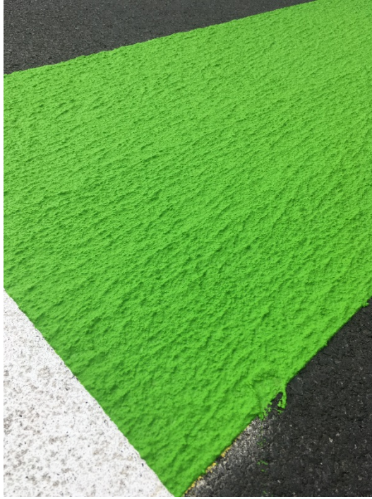
Figure 17: Close-up of curing CycleGrip MMAX
