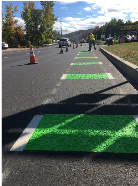
Figure 43: Finished Transpo Color-Safe Bike Lane Blocks Near VW Dealership
