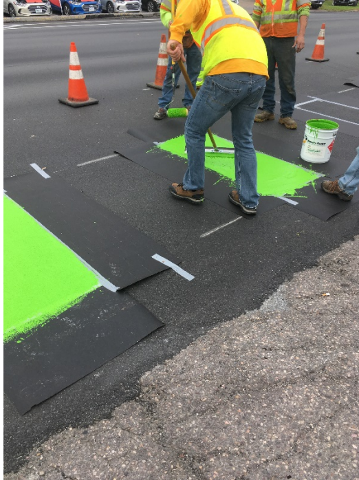
Figure 13: Installation of Ennis-Flint CycleGrip MMAX at the Vermont Shopping Center Intersection
