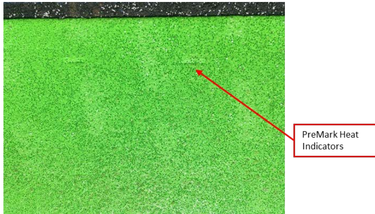
Figure 9: Close-up of PreMark Bike Lane Green showing Heat Indicators
