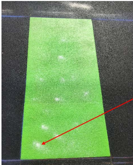
Figure 5: Installed PreMark Bike Lane Green with anti-skid Corundum
