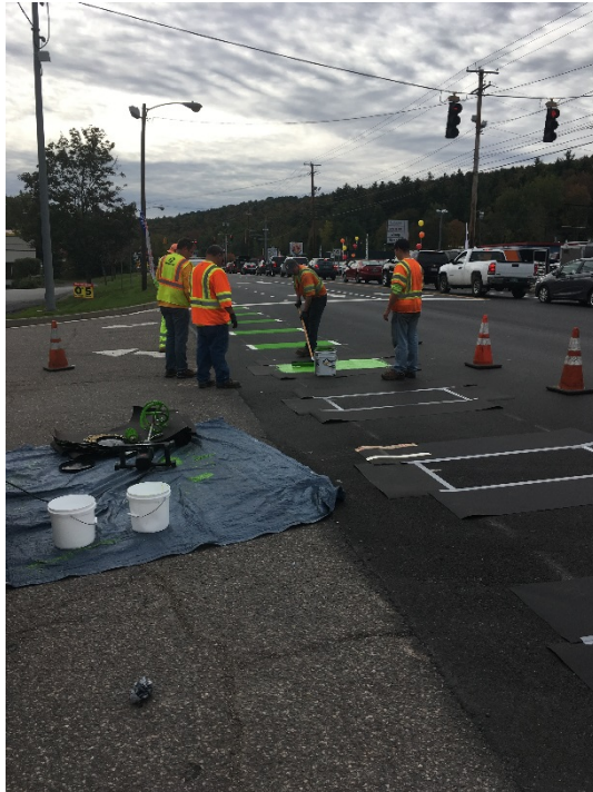
Figure 15: Application of Ennis-Flint CycleGrip MMAX at the Vermont Shopping Center Intersection
