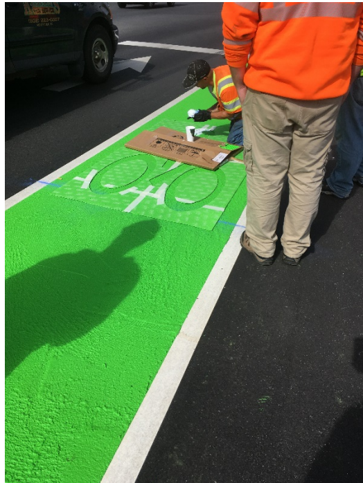
Figure 39: Application of White Color-Safe Biker Symbol at CVS Intersection
