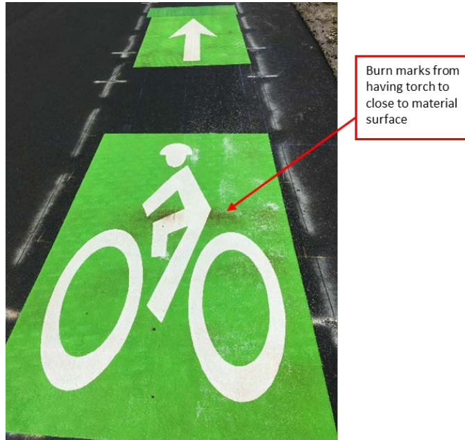
Figure 8: Installed PreMark Bike Lane Green Biker Symbol
