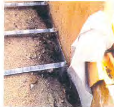
Figure 7. Reinforcing Strip Connection
