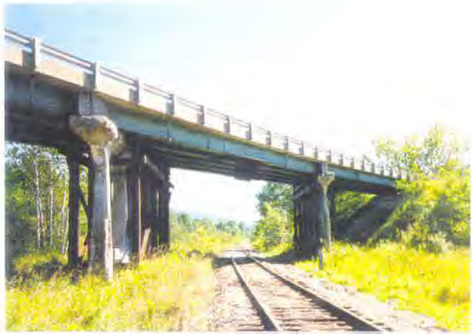
Figure 1. I-Beam Bridge, Constructed 1937
