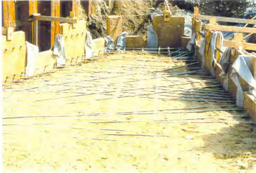
Figure 4. Acute Corner Reinforcing Strip Layout
