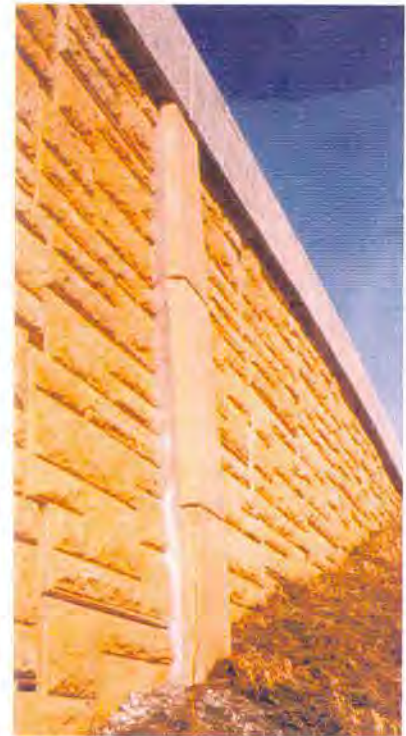
Figure 8. Repaired Slip Joint Wingwall 4
