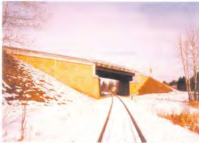
Figure 16. Completed MSE Abutment Walls
