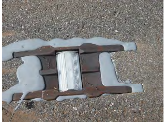
Figure 2 – Marker in Place with Epoxy
