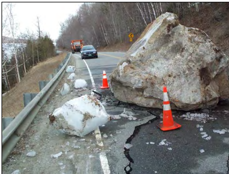
Figure 1 Rockfall on VT Route 5A in Westmore, Vermont
