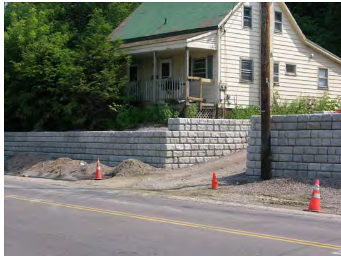
Figure 5: Retaining Walls 1 and 2 constructed with a 90° turn.
