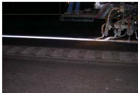
Figure 4- White line being applied
