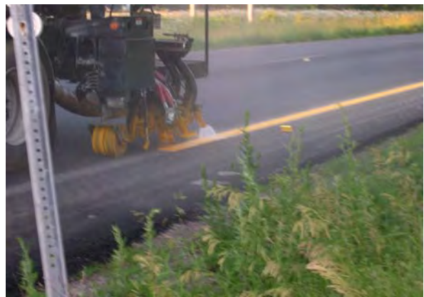
Figure 3- Yellow Edge line being applied (MM 0.55 WB)
