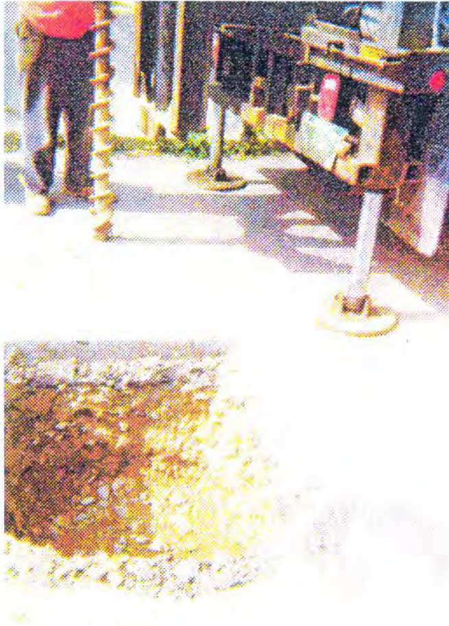
Monitoring well installation at field permeability testing
