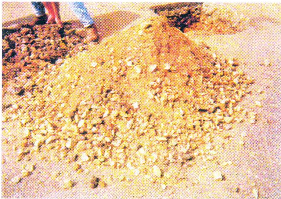
Large-scale field permeability test on dense graded crushed stone
