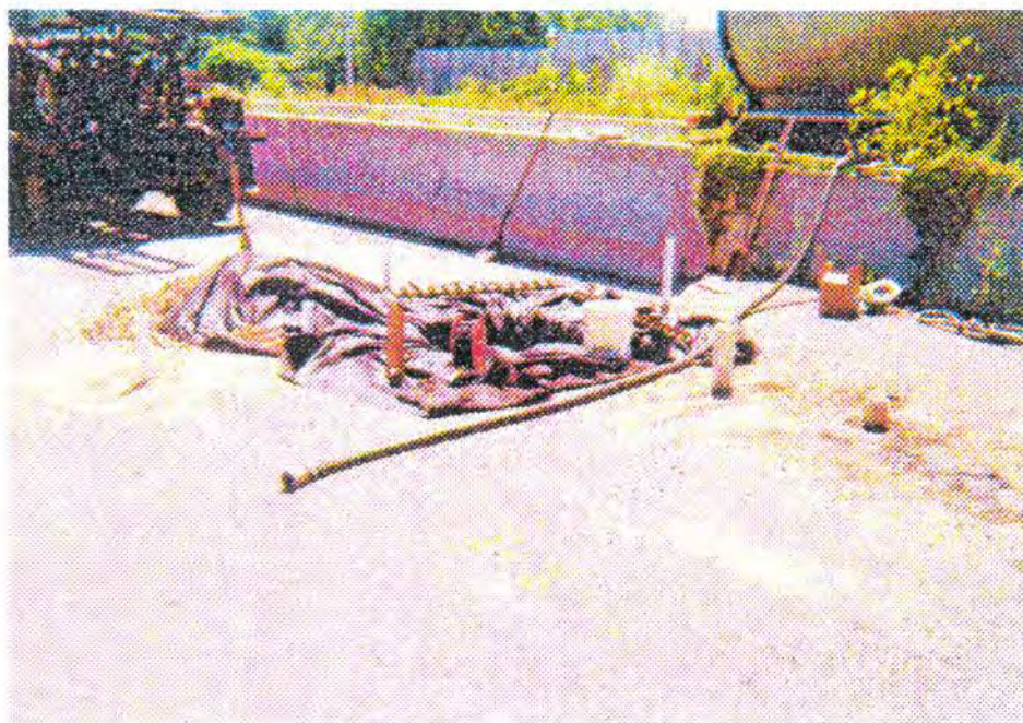
Monitoring well array and experiment setup for field permeability test
