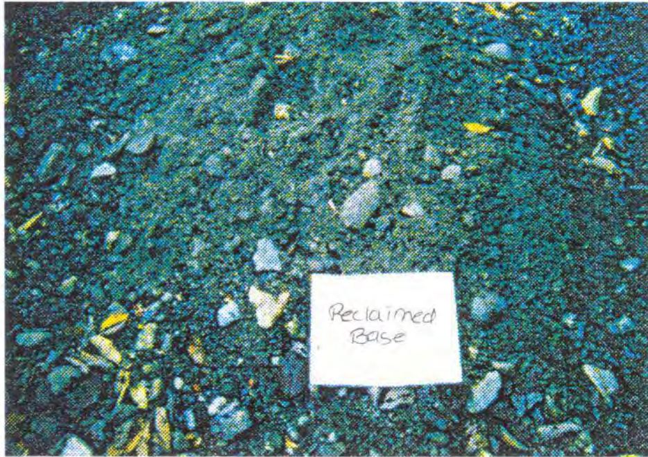
Reclaimed base provided by VAOT from Route 140, Mount Holly, VT
