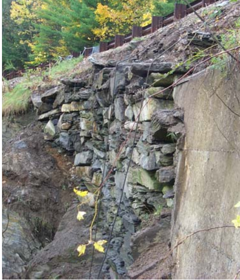
Figure 3: Laid up masonry wall, immediately west of slide area.
