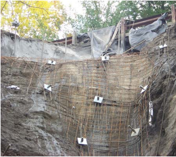
Figure 9: Welded wire fabric and rebar on mortared masonry wall.
