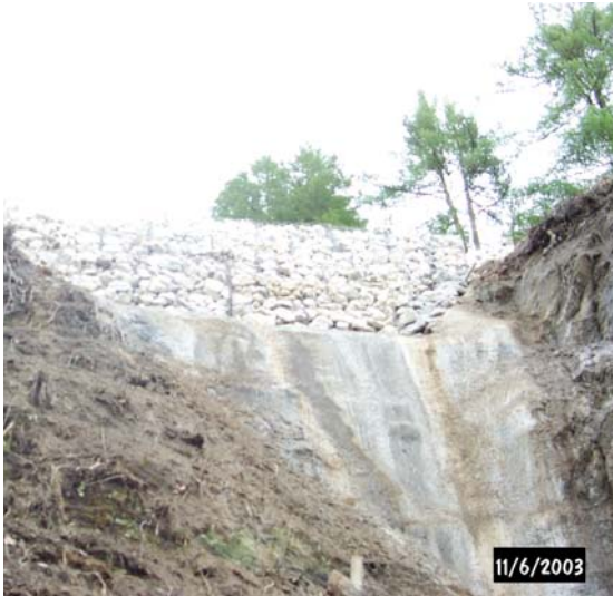
Figure 11: Completed repairs to mortared masonry wall below slide area.
