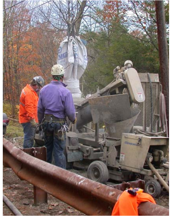
Figure 6: Shotcrete pump with a bag of shotcrete suspended over it.
