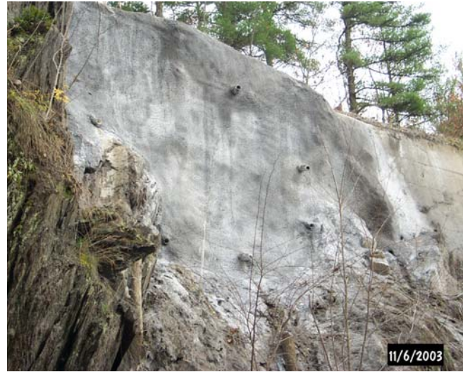
Figure 12: Completed repairs to laid up masonry wall.
