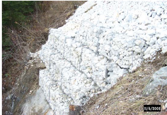
Figure 10: Completed Gabion wall
