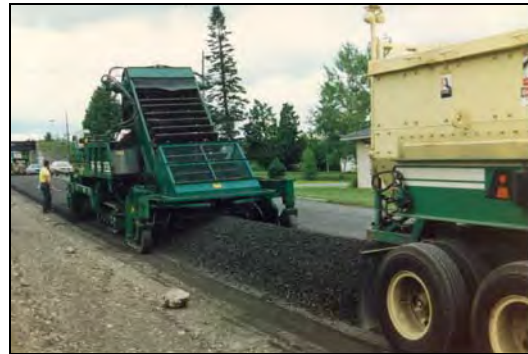
Figure 2 – Recycle Train Mixing Unit/Paver
