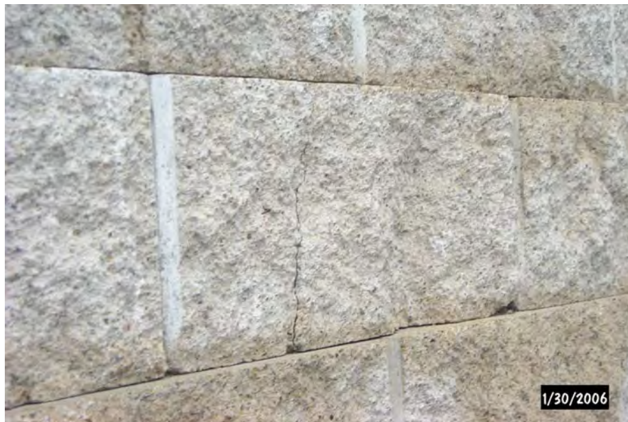
Figure 8b – Vertical fracture
