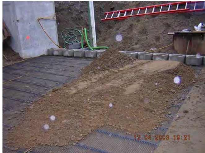
Figure 1: Geogrid being placed in layers of compacted fill.
