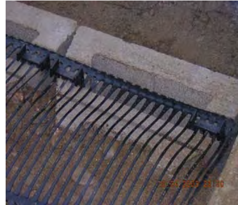
Figure 5: Clips installed through geogrid into modular block.
