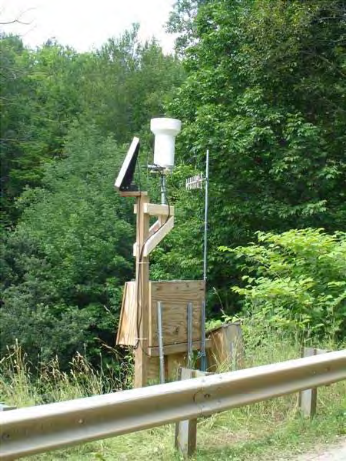
Figure 3.7 Installed rain gauge.
