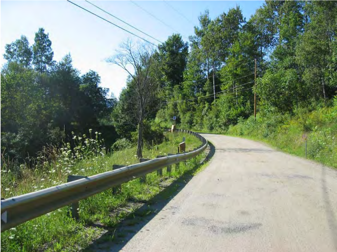
Figure 3.2 General site layout, with Inclinerometers 1 & 2 in the foreground and Inclinerometer #3 and the data acquisition system in the background.
