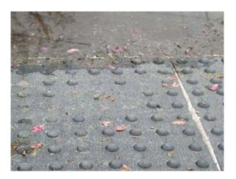
A number of domes have been completely removed. Based on the overall condition of this product only 3 years after installation, it will be recommended to remove it from the Approved Products list.
