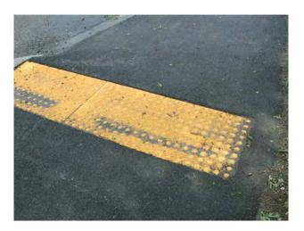
It was noted on one of the panel installations that a void had formed under the panel, allowing it to deflect when stepped on. Installation of these panels on asphalt must be done carefully to avoid such voids. Continued deflection may cause the panel to crack over time.
