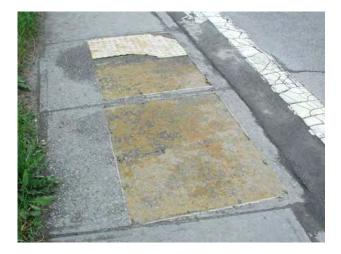
This flexible product experienced almost complete removal after being exposed to one winter of sidewalk plowing, demonstrating a poor bonding to the underlying concrete.
