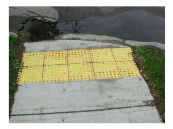
At least 50% of the domes have been lost or severely damaged. The overall condition is fair to poor. The tiles are intact and have not separated from the surrounding concrete.
