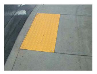
The overall durability of this product is very good. An early installation showed problems with the coating that is adhered to the stainless steel panel. The product in place incorporates a new coating process and small ridges on the domes that are intended to cause any plow blades to ride above the normal dome top.
