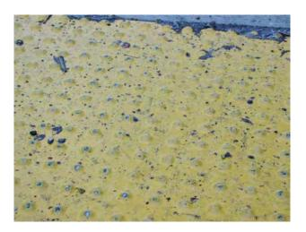
The removal of surface coating was noted on some internal domes, not just the leading edge.
