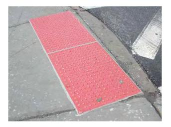
The overall condition and appearance of this product is very good. Color has not significantly faded since its original installation. Joint seams are intact.
