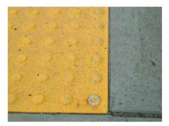
Some of the small ridges had been removed by the plow and there are signs of complete removal of the coating, exposing the underlying stainless steel. One dome on a leading edge of the panel was partially crushed.
