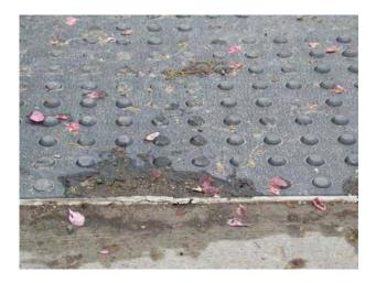
Some small sections of panel have been completely removed and. Many dome show signs of scraping.
