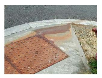
The one feature of this product that will need to be monitored is the extent to which the rust "bleeds" onto adjoining surfaces. Some bleeding was observed on this ramp, but generally was very limited.
