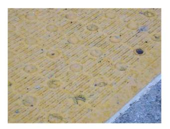
In addition to the wholesale removal of sections of this product, individual domes were crushed and sheared off. This product is considered to have failed.
