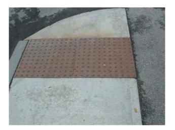
These panels showed virtually no damage and all domes were intact. There was good color contrast to the surrounding concrete. Some minor bleeding of rust onto the adjacent concrete was observed.
