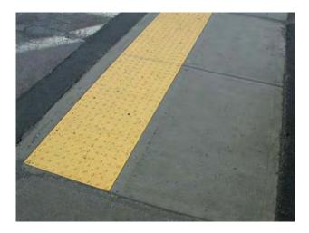
Overall condition of this product is good. There is some damage to the panels. No evidence of separation from underlying concrete.
