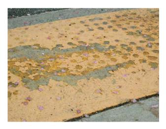
In addition to entirely missing sections, many individual domes have been removed.
