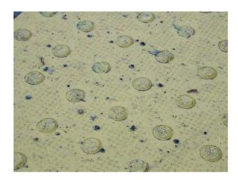
Individual domes are chipped and broken. It is likely that many domes no longer meet the ADA standards for dome height.
