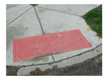
The panel is adhered well in the surrounding concrete. However, at least 50% of the domes have been lost or severely damaged.
