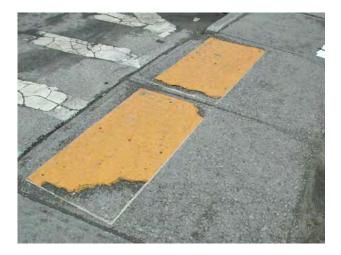
After one winter, the product is showing considerable signs of wear and exhibits a poor bonding to the substrate.
