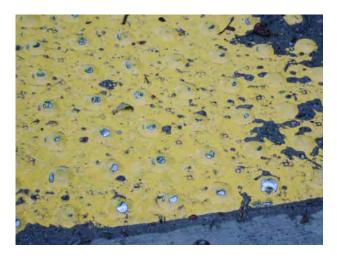
The panel surface is showing the impact of one winter of sidewalk plowing in that some of the coating has been removed from the panel, exposing the underlying stainless steel. Some minor dome damage was present.
