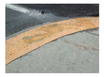
Large sections of the coating have been completely removed from the ramp surface.
