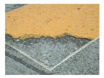
It appears that the sidewalk plow blade lifted one corner of this semi-rigid panel and broke the piece of panel off.
