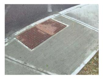
The natural rust color of these panels appears to provide adequate contrast to the surrounding concrete, even when the concrete is wet.
