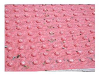
There are a few missing domes and some scraping of dome tops is evident, especially on the leading edge of the panels.
