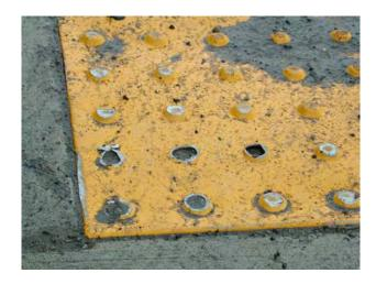
Of most concern with this product is that where complete domes have been removed, a hole in the panel surface has resulted. This will allow water to accumulate under the panel surface and may cause problems when subjected to the freeze-thaw cycle. It is likely that this product will not be recommended for use on Agency projects.
