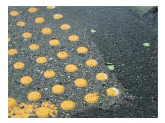
As with almost all products evaluated, the leading edge of the panel is where the majority of damage was observed.
