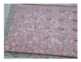
Approximately 25% of the domes show signs of chipping or crushing as a result of winter maintenance. It is expected that continued deterioration would take place with this product.
