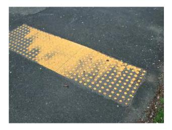
Sand and gravel from the adjacent road and winter maintenance had accumulated between the domes on portions of the panels. The panels were in very good shape overall.
