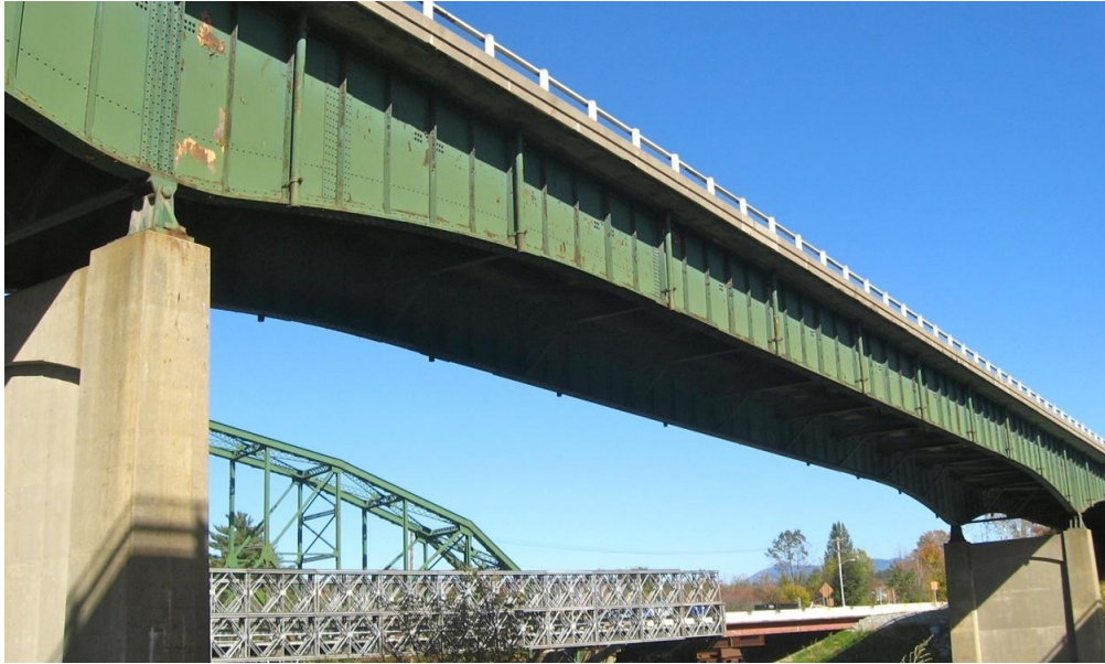
Figure 2.2: Overall view of bridge 58N from Winooski river
