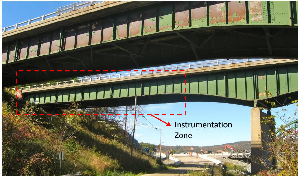
Figure 2.7: Instrumentation zone in Bridge 58 North
