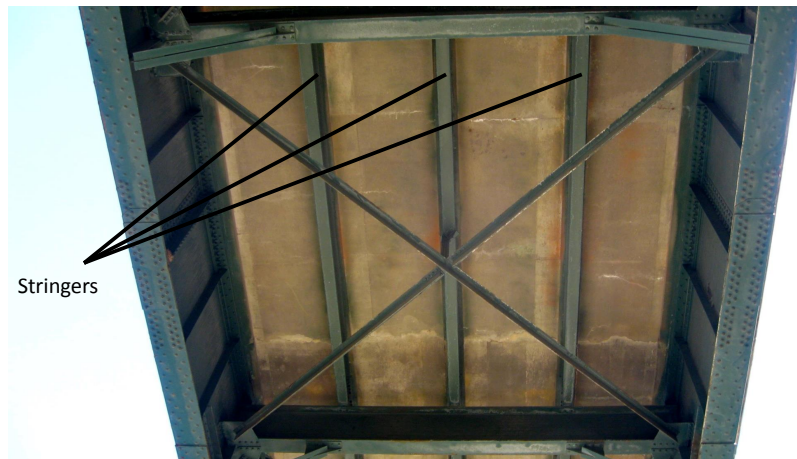
Figure 2.3: View of underside of bridge deck with stringers indicated.
