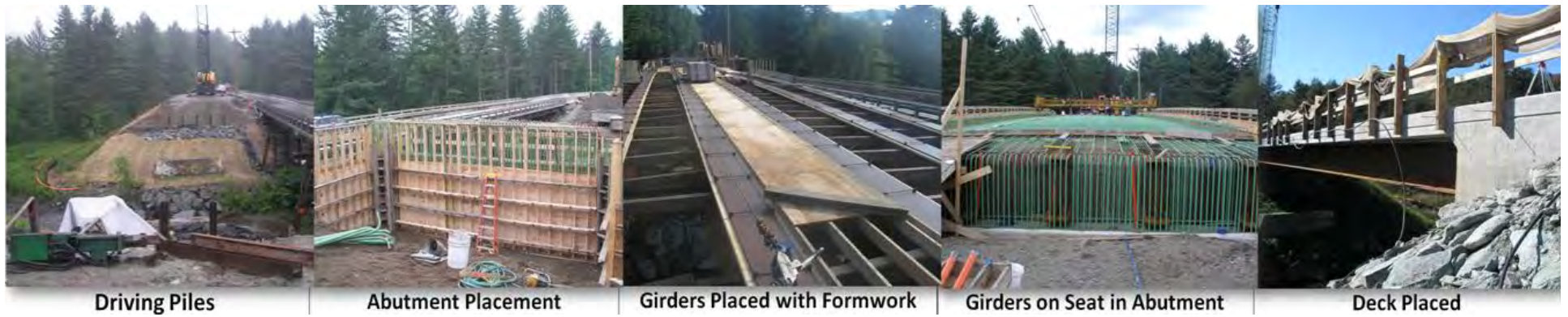
Figure C-0-4: Middlesex Bridge Construction
