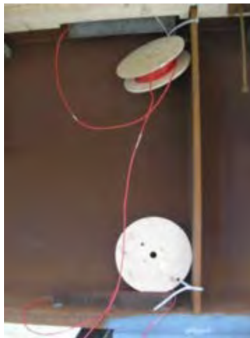
Figure 3-40: Girder Strain Gages on Top and Bottom Flanges with Protective Angles
