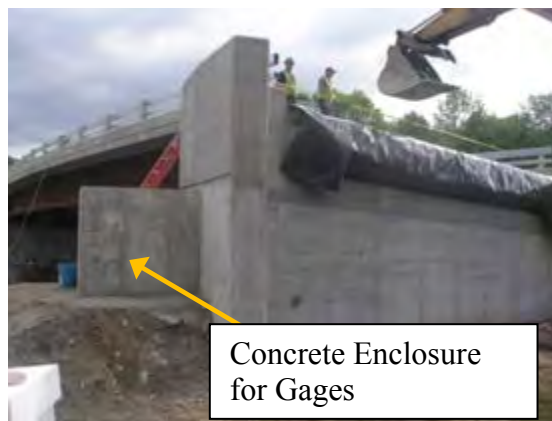
Figure 3-46: Displacement Transducer Enclosure
