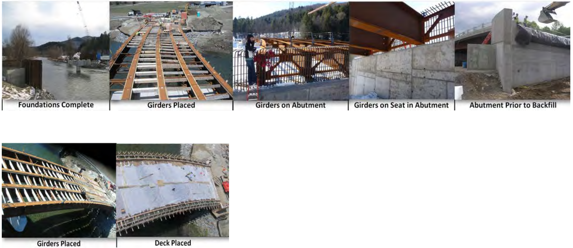
Figure C-0-6: Stockbridge Construction
