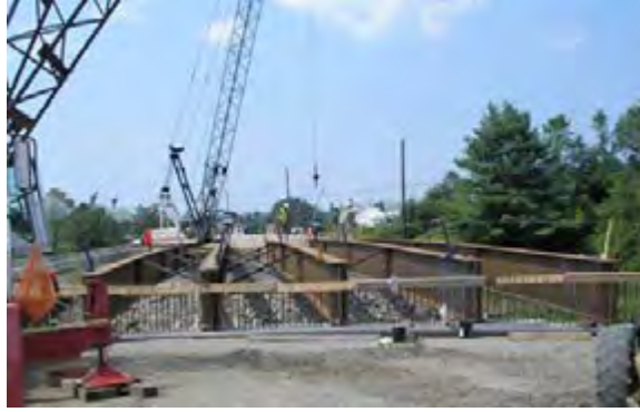
Figure 7-2: Girders Placed at the East Montpelier Bridge
