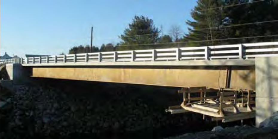
Figure 2-6: East Montpelier Bridge
