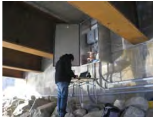
Figure 5-9: East Montpelier Load Testing (Data Acquisition during Testing)
