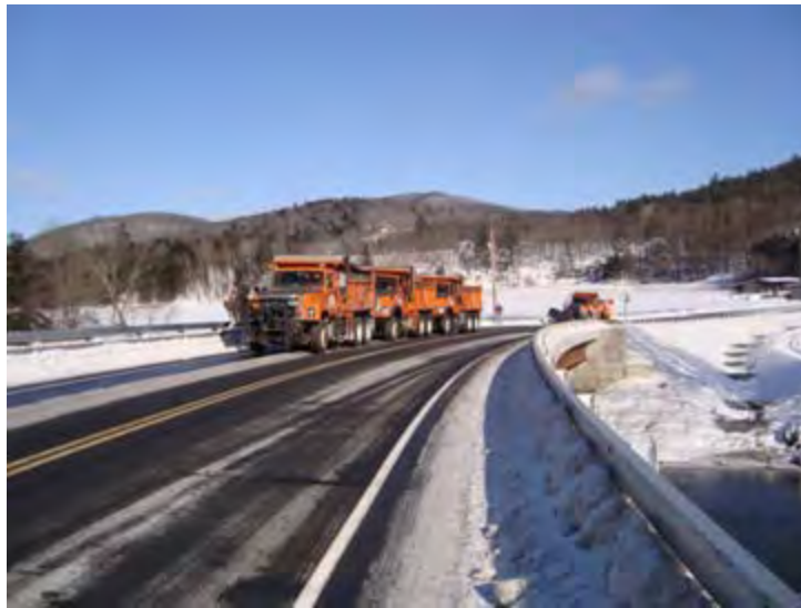
Figure 5-17: Stockbridge Bridge Load Testing
