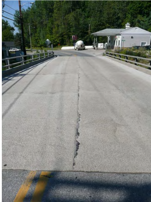
Figure 17 Application after installation in 2008
