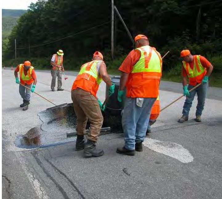
Figure 8 Placement of the second lift.
