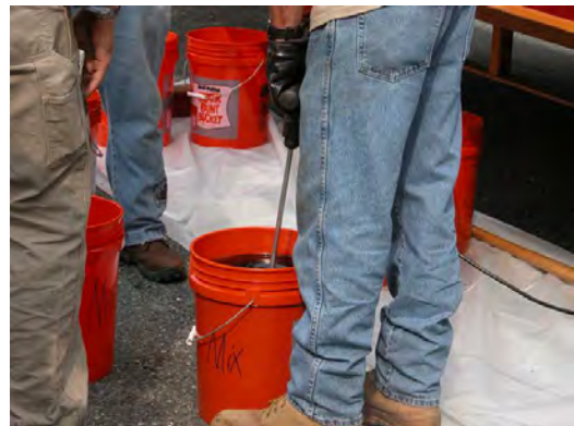
Figure 5 Mixing the Epoxy
