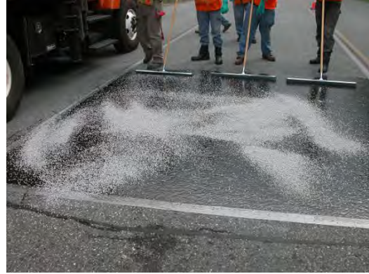
Figure 7 Spreading limestone
