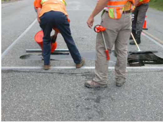
Figure 6 Spreading Epoxy
