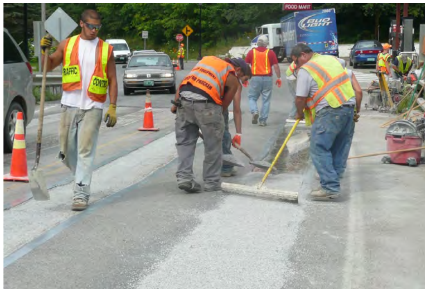
Figure 20 Repairing the wheel paths.
