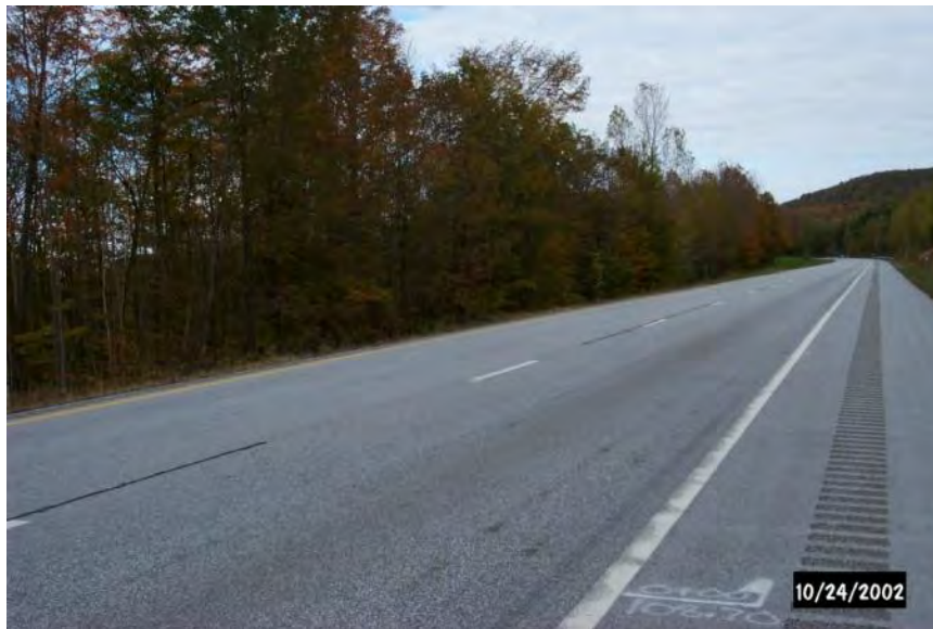
Figure 4 Typical Control Site (MM 108.70)
