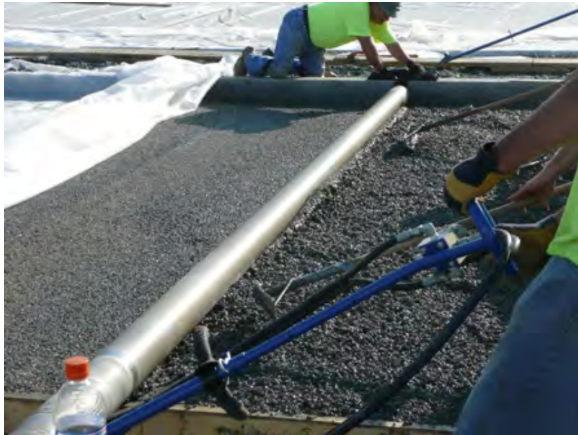
Figure 3. Placement and rolling of porous concrete.
