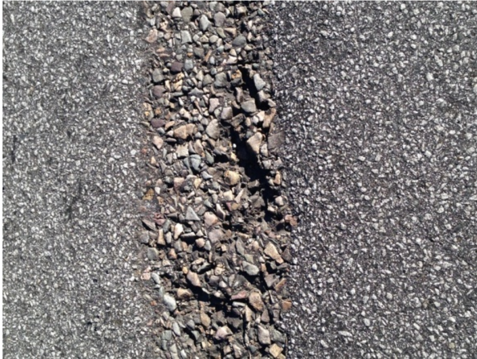
Figure 25: Pavement wear.
