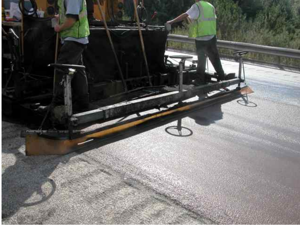
Figure 4: Slurry Seal paving.
