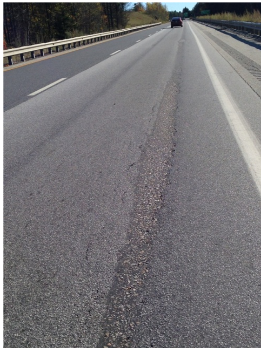
Figure 24: Thin HMA Overlay section overview, just prior to paving in 2013.
