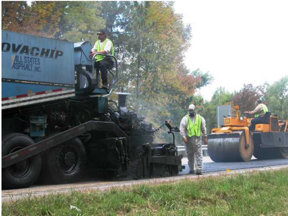
Figure 6: NovaChip® paving.
