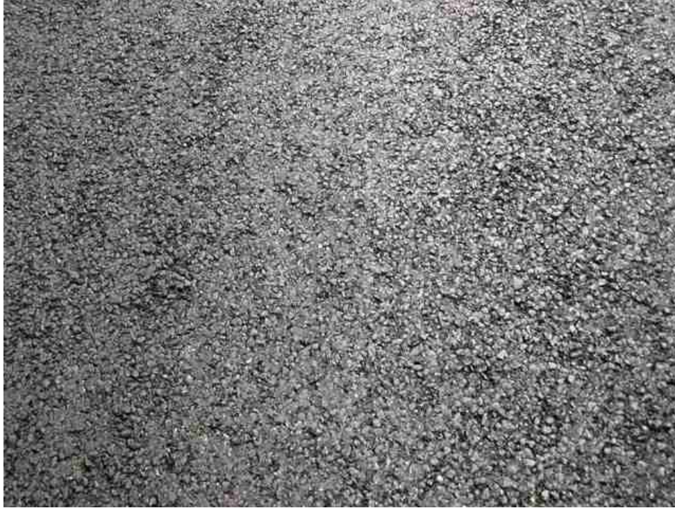
Figure 7: Completed NovaChip®.
