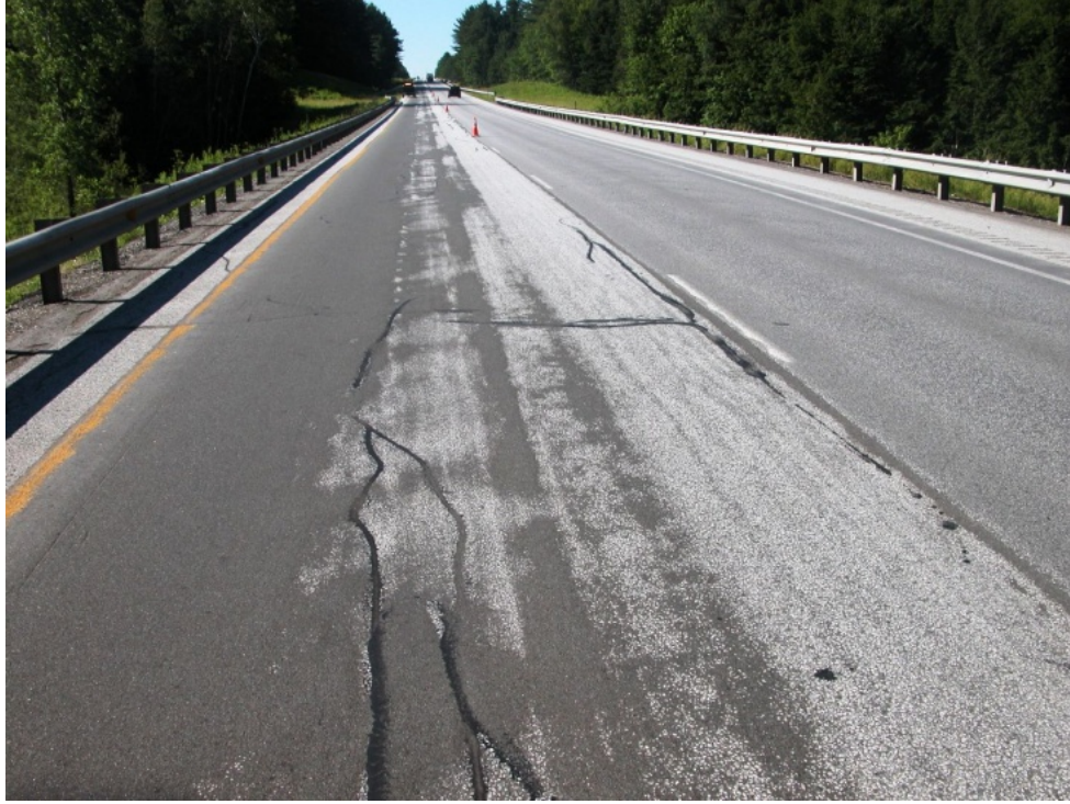
Figure 16: 2007 Slurry Seal and Thin HMA Overlay overview.
