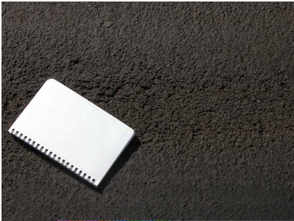
Figure 5: Completed Slurry Seal.
